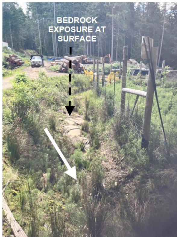
Photo 6. Drainage ditch along north side of roadway looking westerly, May 20, 2025. White arrow indicates drainage flow direction.
