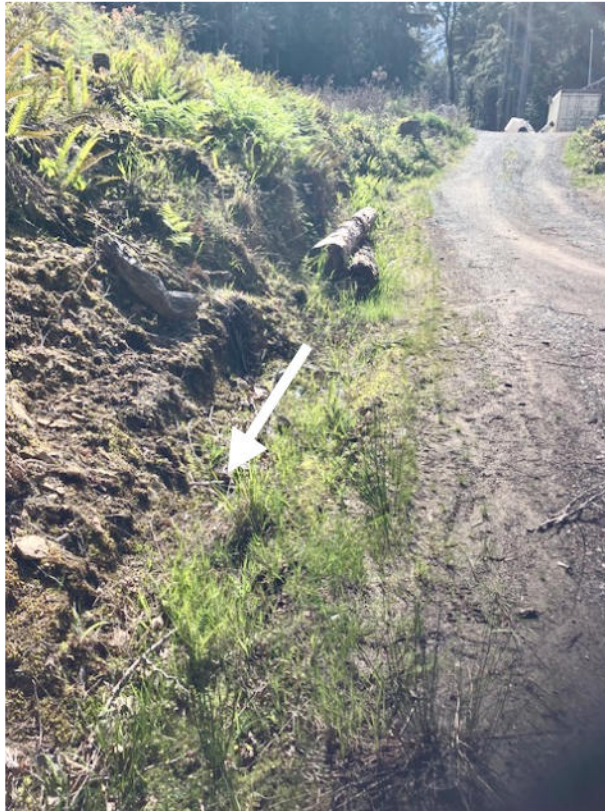
Photo 5. Drainage ditch along south side of roadway looking westerly along southern side of property, May 20, 2025. White arrow indicates drainage flow direction.
