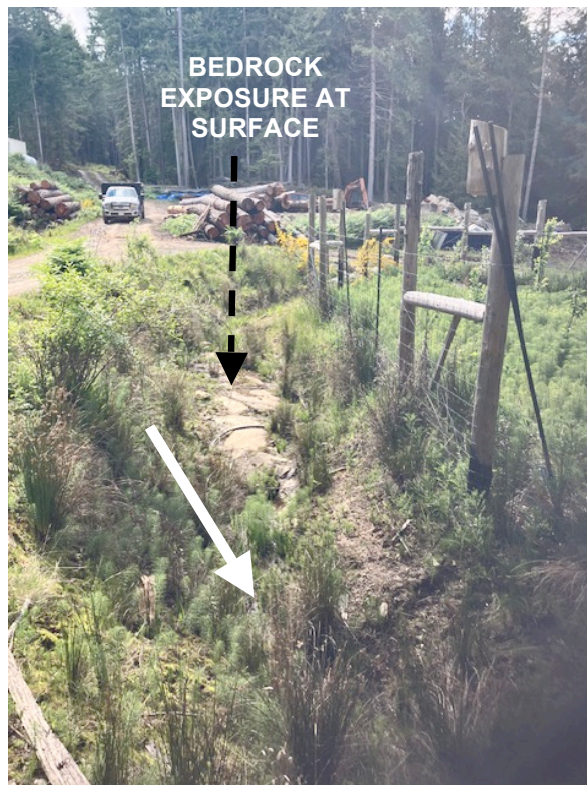
Photo 6. Drainage ditch along north side of roadway looking westerly, May 20, 2025. White arrow indicates drainage flow direction.
