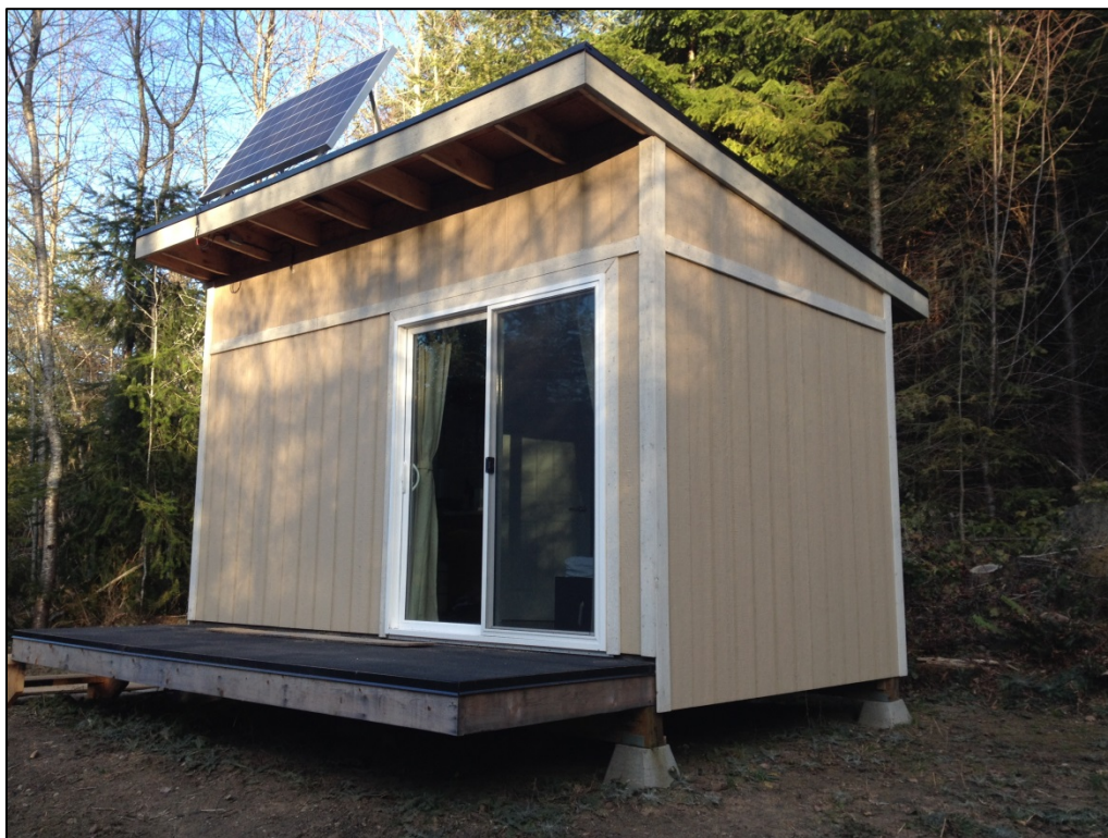
Picture 4: Newly constructed meditation hut on Lot A
