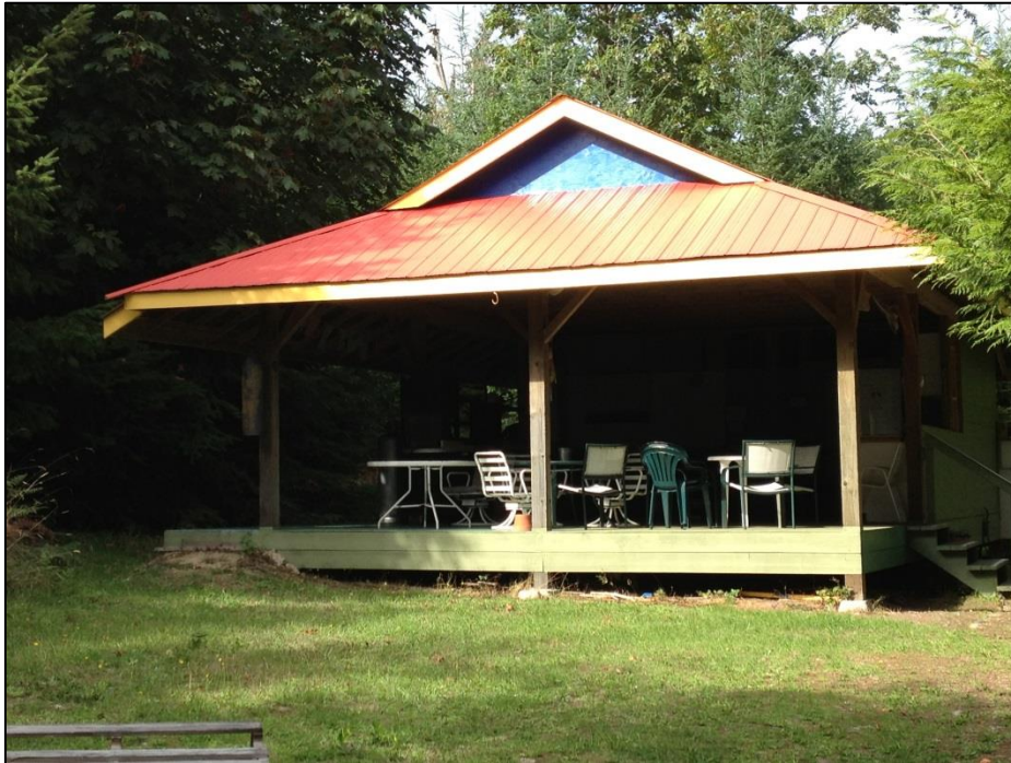
Picture 1: Outdoor Kitchen (on Lot A)
