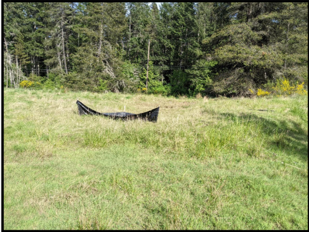
Photo 29 – Silt fencing placed within swale that acts as overflow discharge for reservoirs. Fencing showed little to no evidence of siltation occurring as a result of stormwater discharge to ditching.
