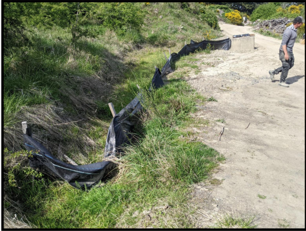
Photo 25 – Silt fencing in place parallel to Site ditching and access road appears to have been functioning well over the rainy season.
