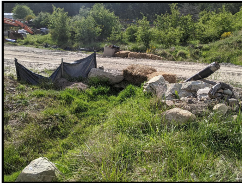
Photo 26 – Silt fencing and hay bales in place at ditch crossing.
