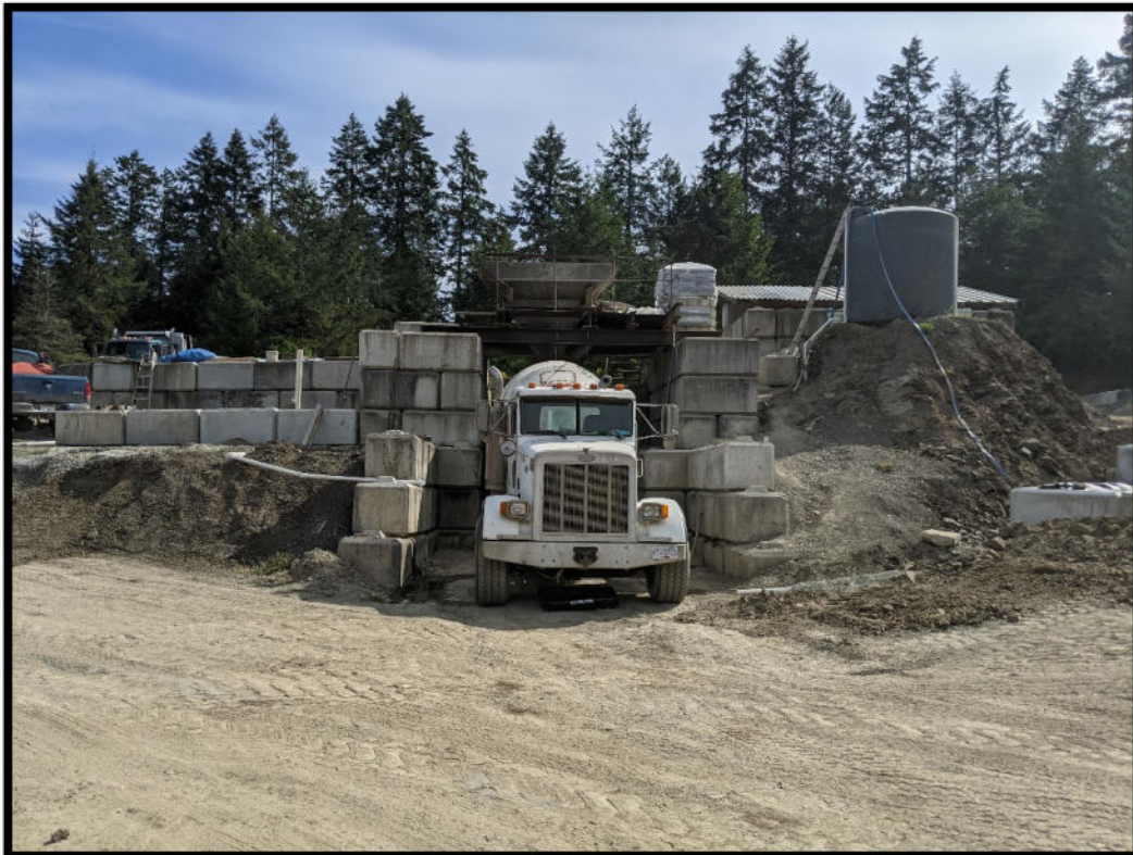
Photo 16 – Drip trays beneath concrete truck in batch plant bay.
