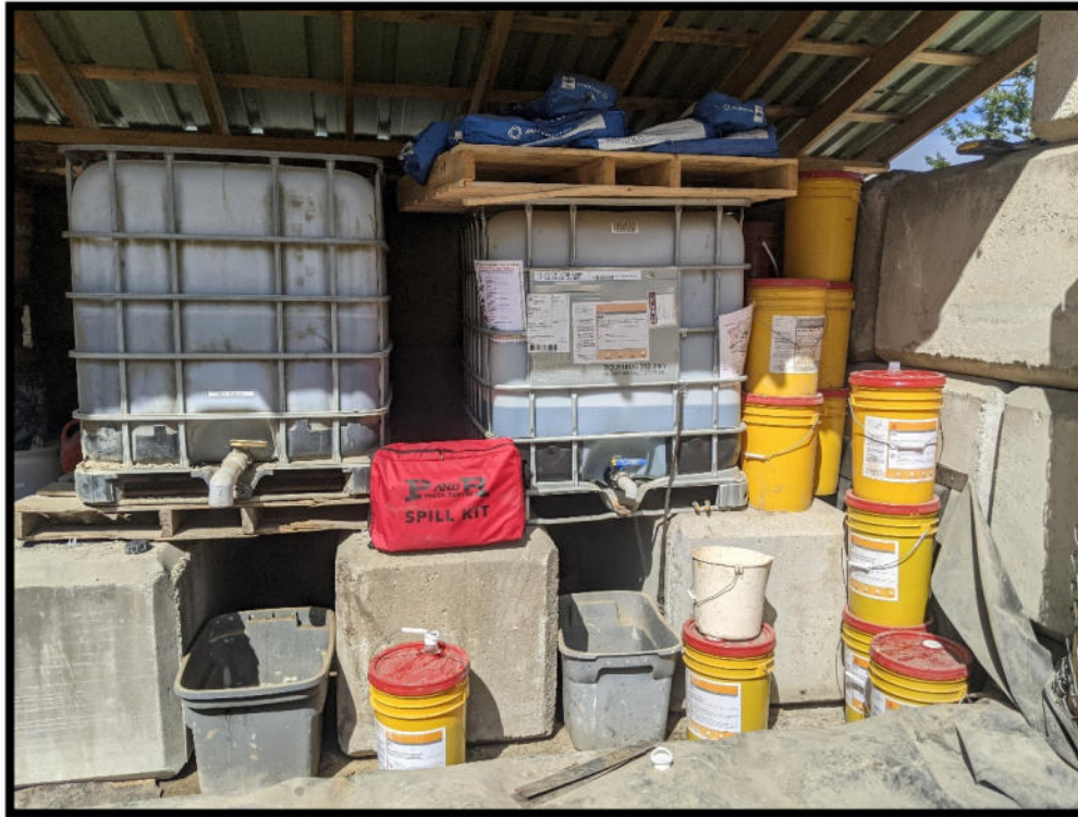
Photo 5 – Interior of chemical storage shed includes concrete additives (stabilizer & water reducers). The shed is lined with 45 mil poly liner as a means of secondary containment. Note spill kit and spill response plans posted on 1000L totes.
