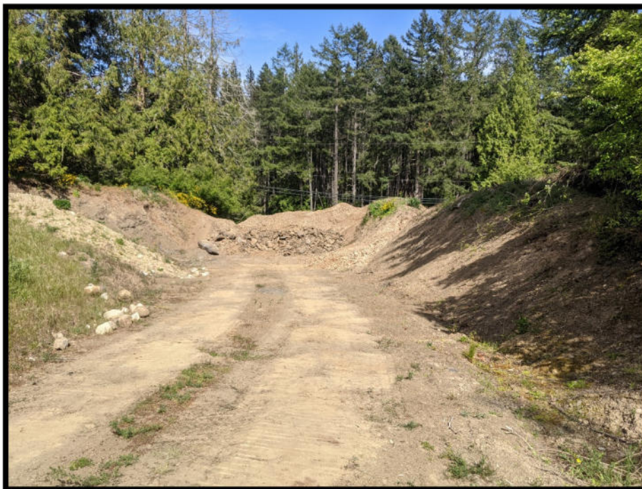
Photo 2 – Current progress of proposed Site Access 'A'.
