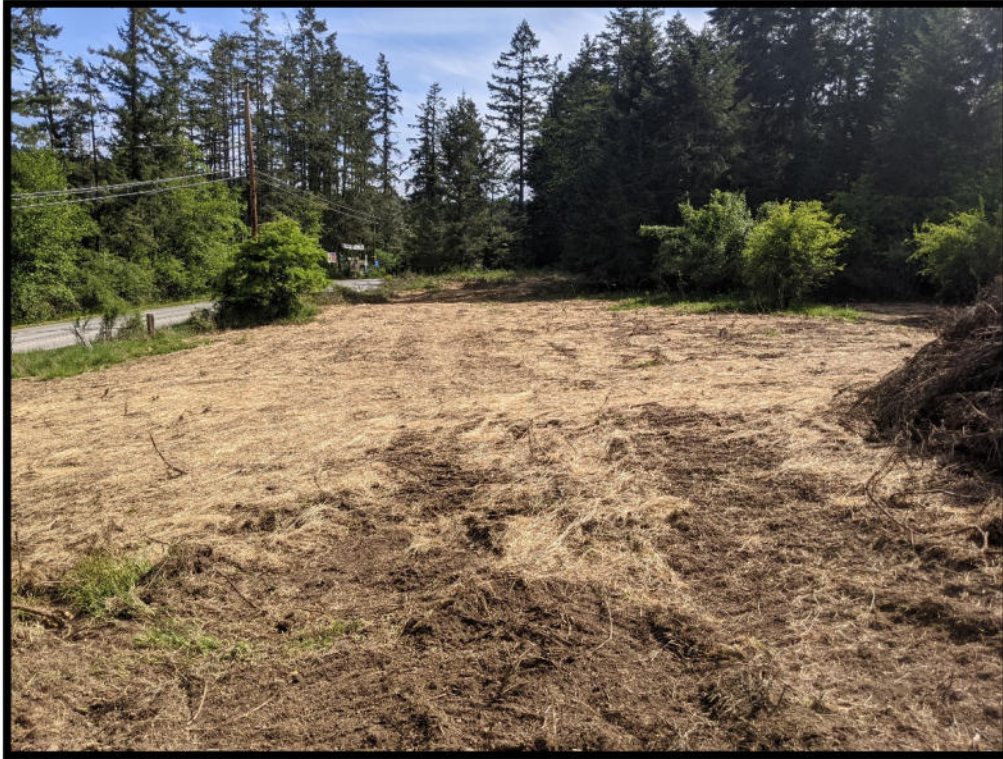
Photo 3 – Natural grassed area, south of Site Access ‘A’. Vegetation has been cleared and seeded, exposed ground is covered with hay as a means to prevent erosion.
