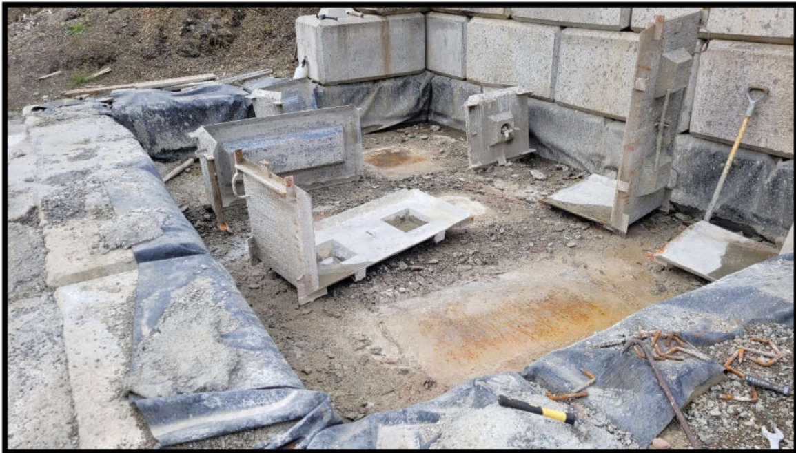
Photo 8 – Poly lined lock block fabrication cell.
