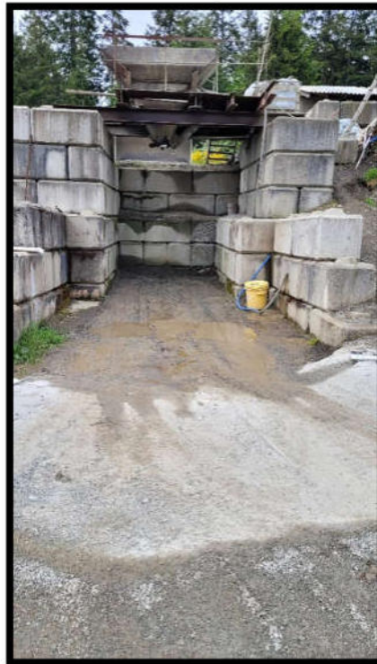
Photo 6 – Concrete batching area with enlarged concrete apron.
