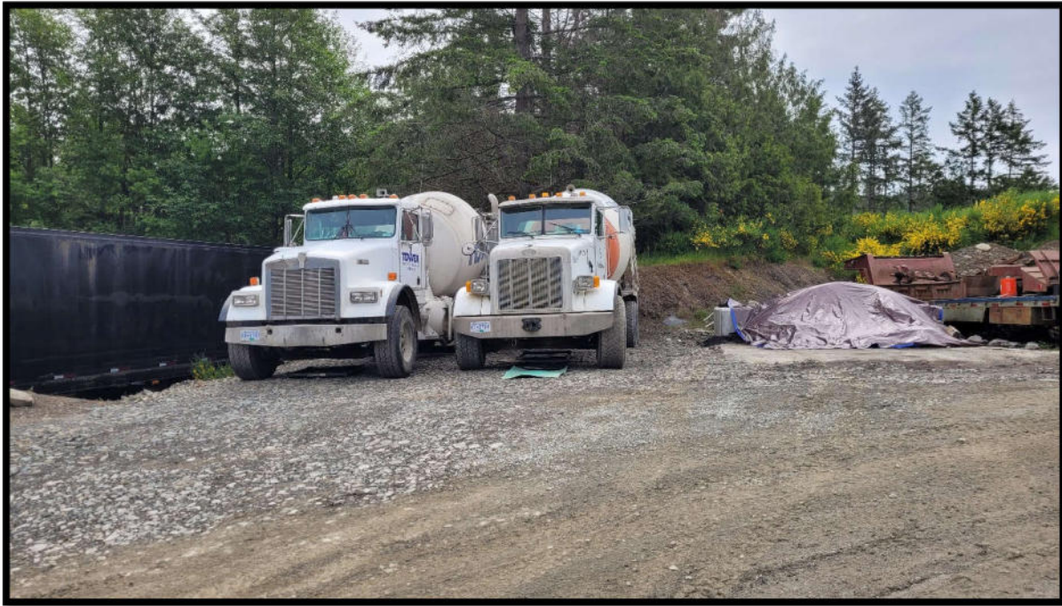
Photo 13 – Parked trucks with spill trays and covered stockpile.
