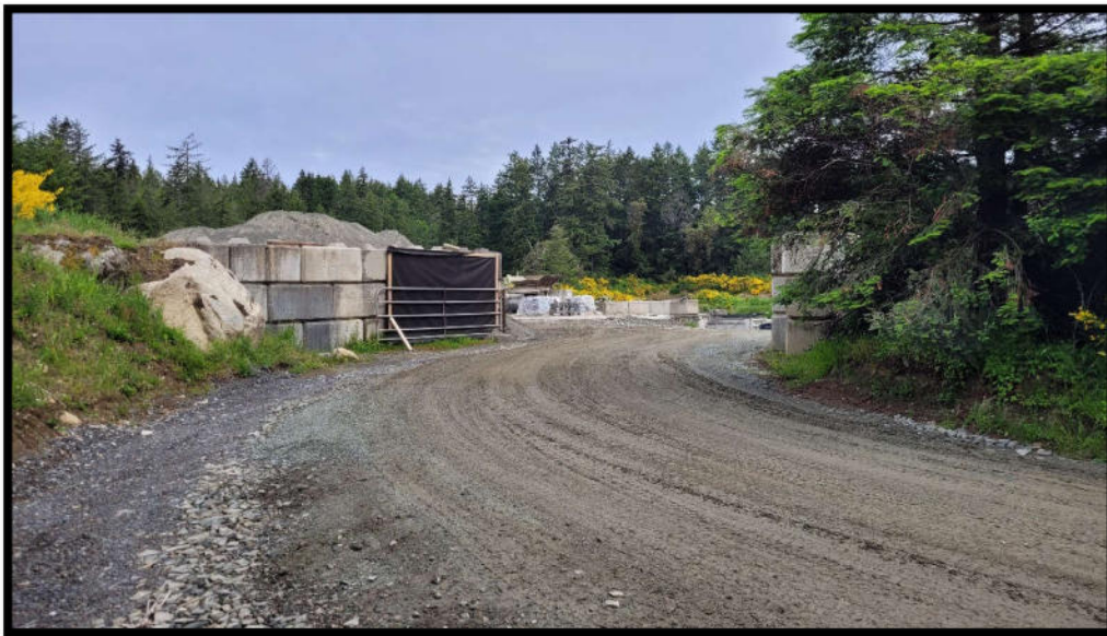
Photo 4 – Lockable gate at site entrance.
