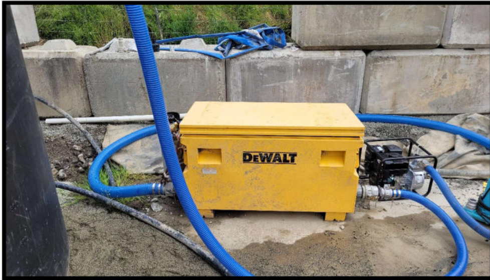
Photo 9 – Water treatment module including pH treatment.
