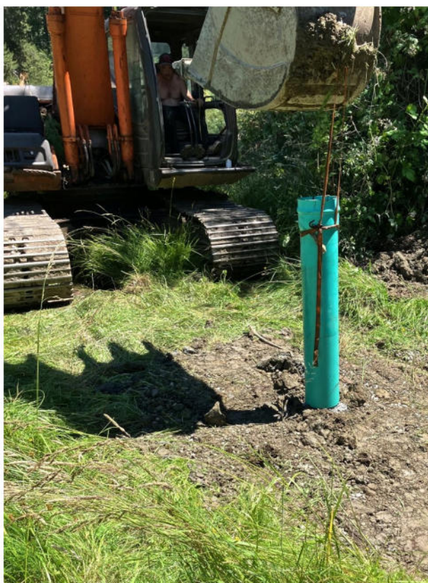
Photo 8. Pulling out 8 inch temporary surface casing, June 30, 2025.
