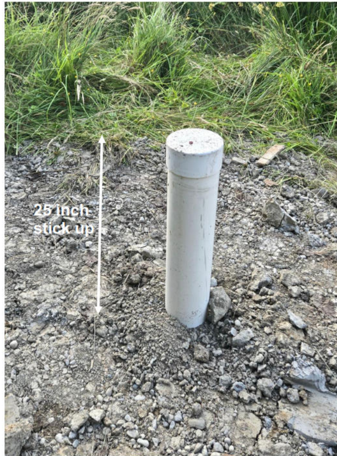
Photo 9. Completed 6 inch diameter monitoring well, June 30, 2025.
