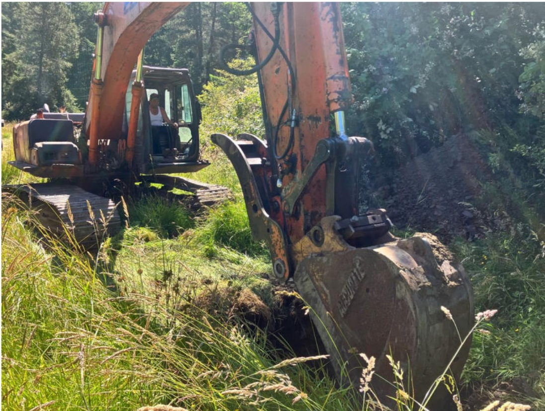
Photo 1. Excavator employed to install monitor well, June 30, 2025.
