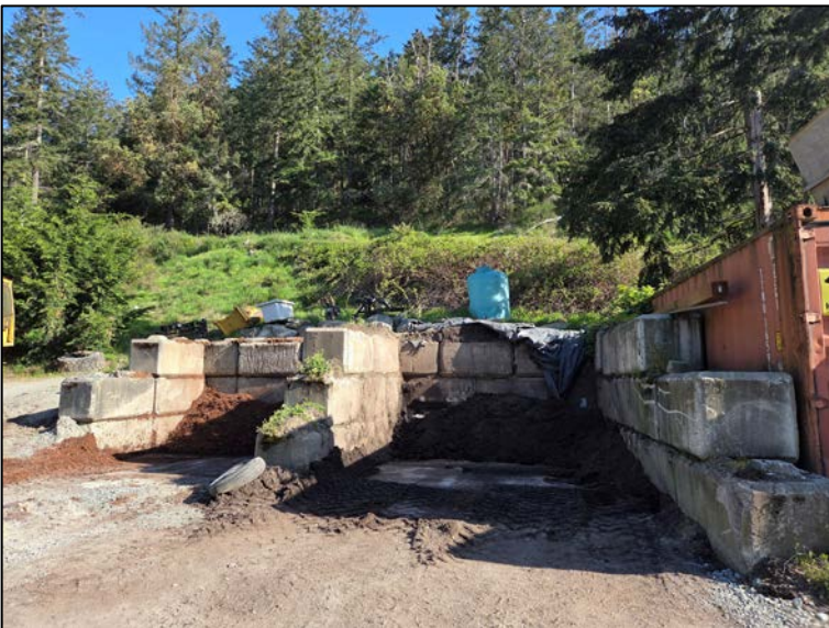
Photo 3: Soils are contained in lock block bins.
