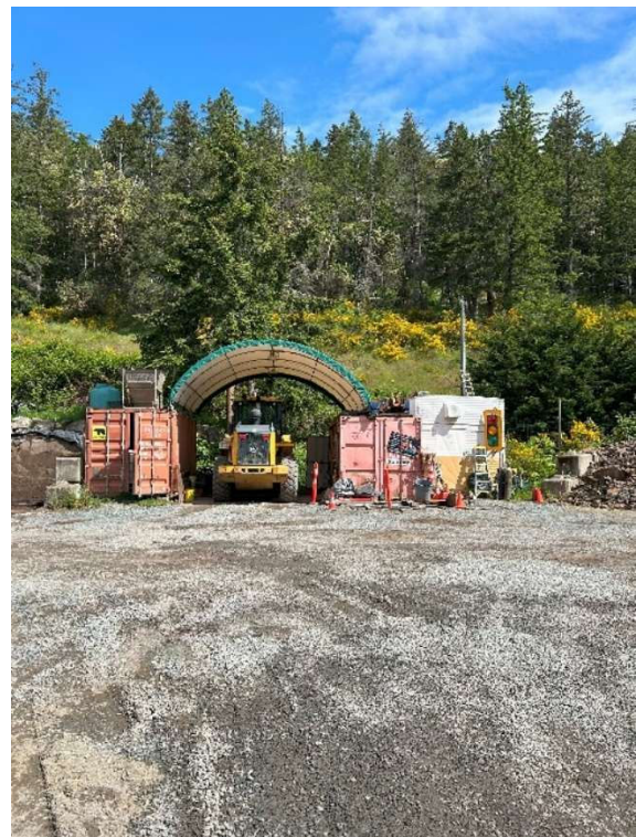
Figure 2: Site Photo Looking North
