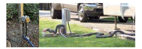
Connecting electricity and water is best serviced with a **service connection node**. The node, typically a wooden post, holds both the water spigot and the electrical plug for the
