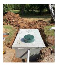
A holding tank is a large sewage container used to collect and temporarily store sewage from an RV. The sewage collected in the container is then removed and transported to an approved location for disposal for a fee. A "Permit to Construct" may be issued if the Health Officer is satisfied that the holding tank is adequate to deal with the domestic sewage originating from the RV and the use of the holding tank will not, if a 'Maintenance Plan' is followed, cause a health hazard.
