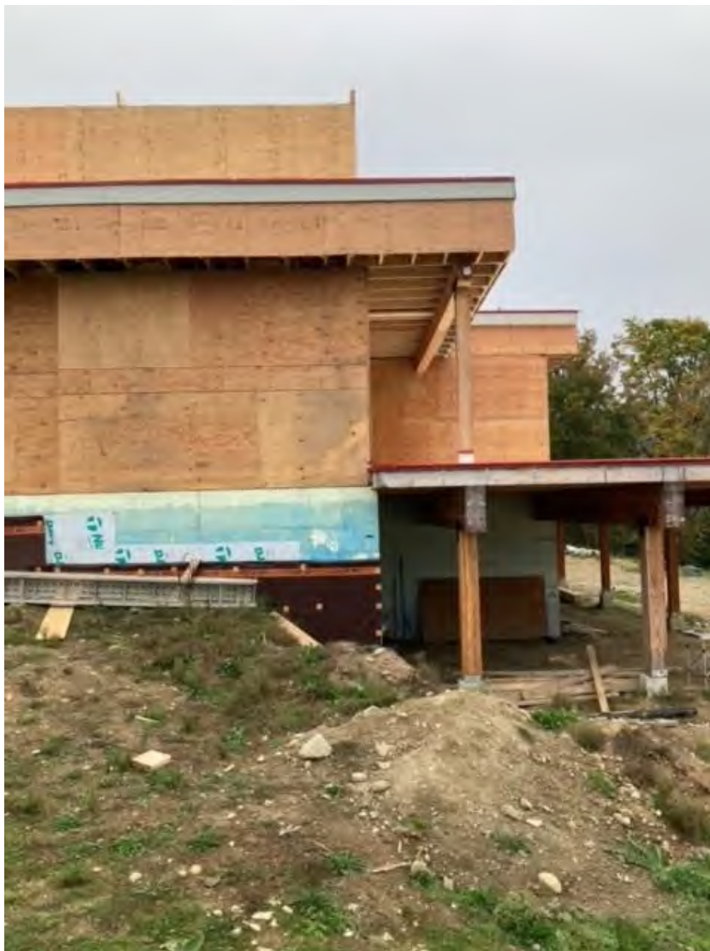
Figure 13 - South East Elevation
