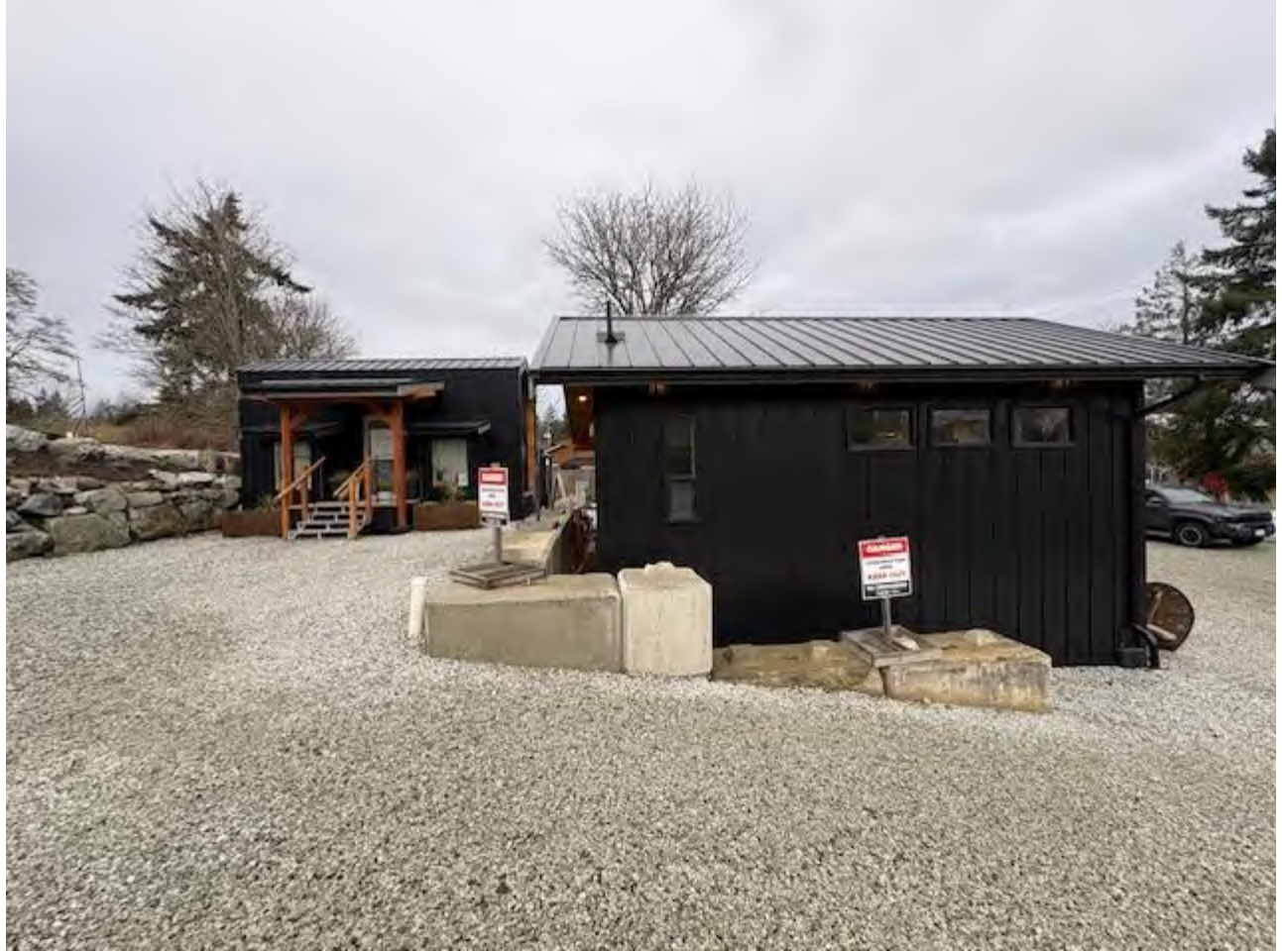
Figure 8 –View Toward North - Building A (Shop) and Building B (Counselling)
