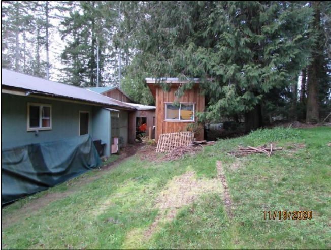
Figure 19: Office area and rear of workshop area behind
