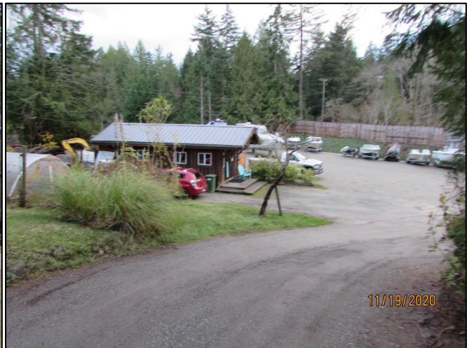
Figure 12: View of home based business building
