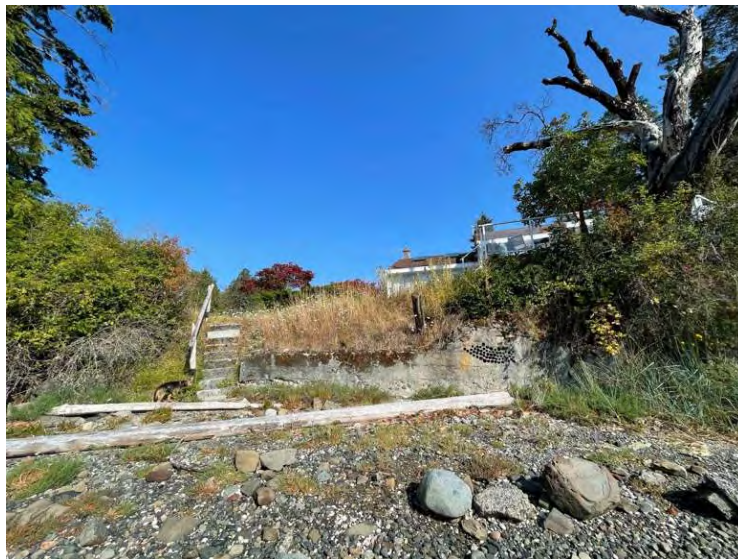
Photo 2. Facing north towards the existing retaining wall.
