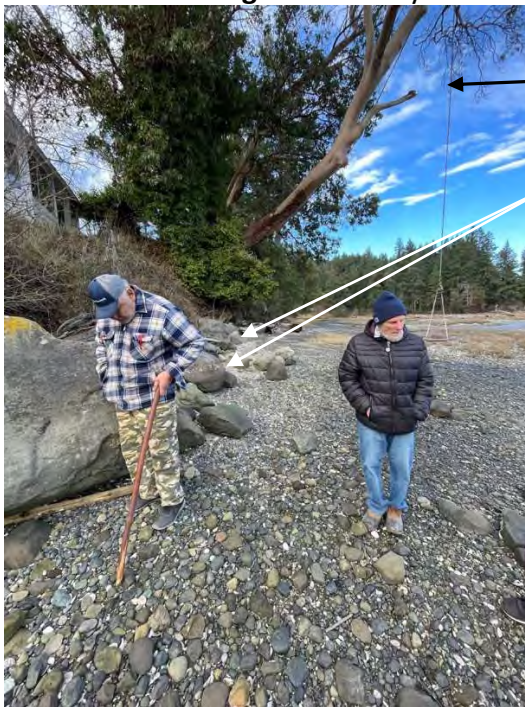
Photo #13. – The Arbutus and swing with the path of large boulders between the white arrows are situated along the E bank in question. 1-3ms between the rocks the existing bank now, so possibly 50 yrs. of erosion?? Photo credit – D. Fenton, Feb 16, 2024.
