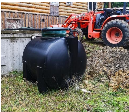
Photos: Common House septic tanks (under construction); Common House
