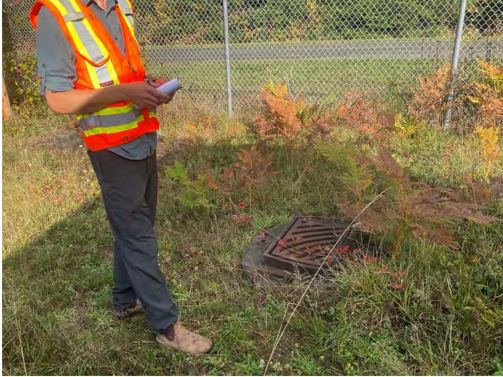
Photo 7. A manhole at the oil-water separator for the vehicle wash pad at the north of the subject lot.
