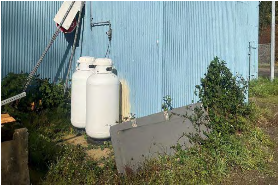
Photo 1. Two propane tanks located next to an office building
