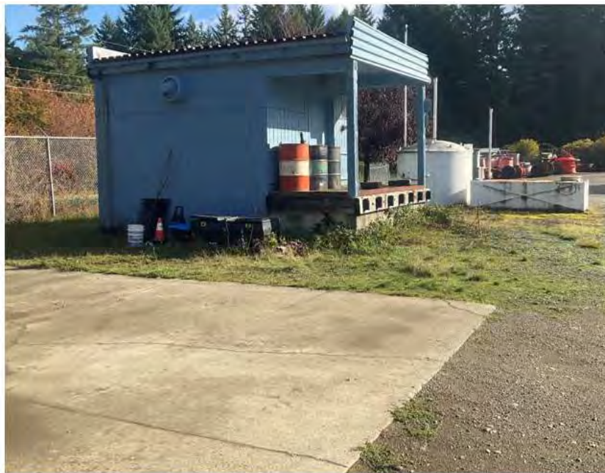
Photo 2. A fuel storage location with a diesel AST and fuel barrels. Vehicle wash pad located in the foreground.
