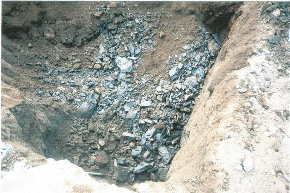
PHOTO 4: Excavation of hydrocarbon-stained siltstone adjacent to former tank nest.
