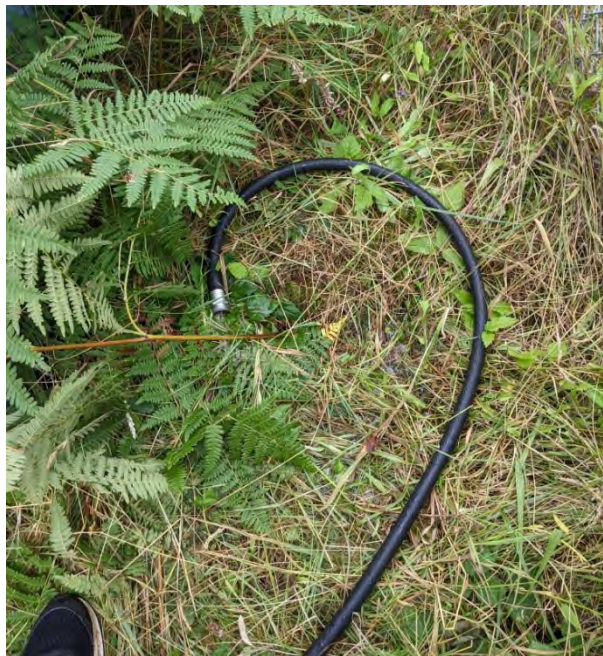
Photo 4. Discharge pipe near the pump house during the 9-day pumping test.
