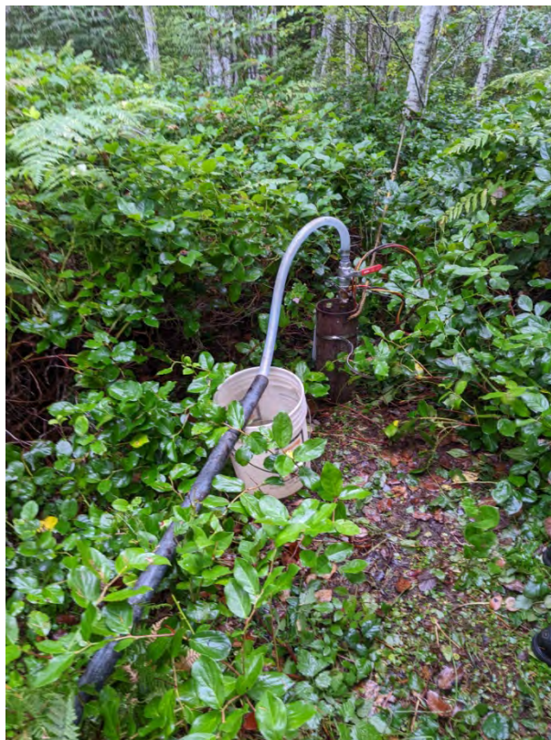
Photo 6. Emcon well with measuring bucket and discharge pipe.
