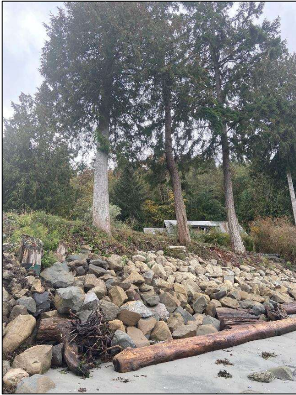
Western portion of revetment at 1160 The Strand
