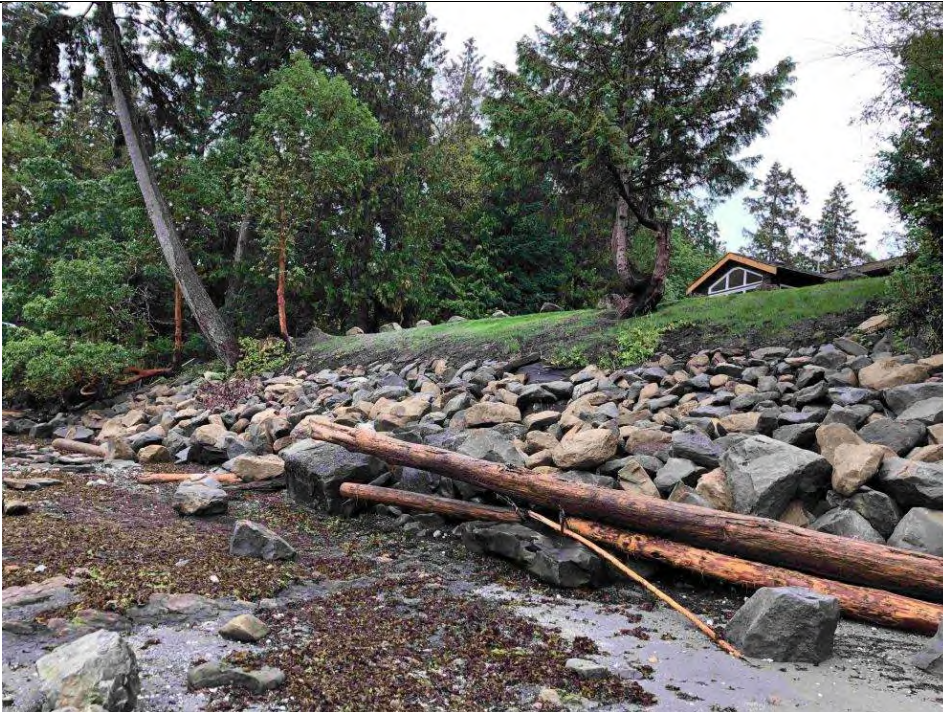
4.) Looking west across subject properties
