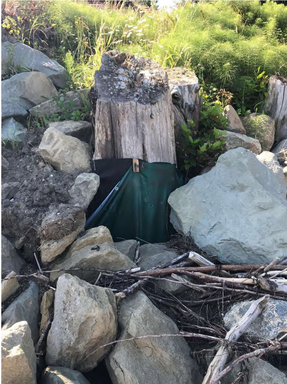
Fig. 7: Evidence of fibre cloth and tarp underlay
