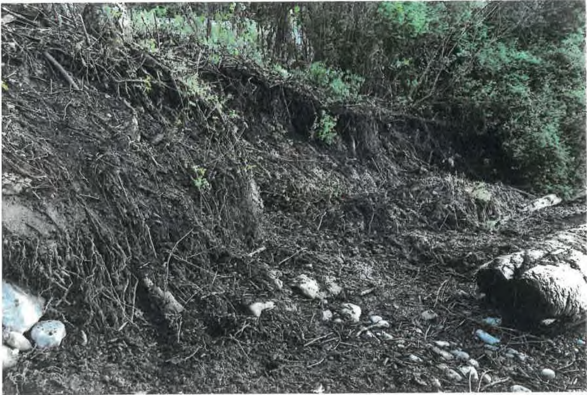
SOFT CLAY AND SOIL BANK SECTIONS ON LOTS THAT WERE BEING ERODED QUICKLY.
