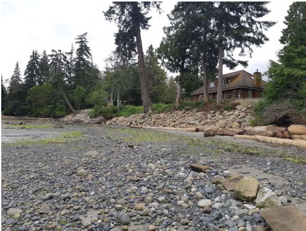
Figure 3.2 Current Shoreline Condition
