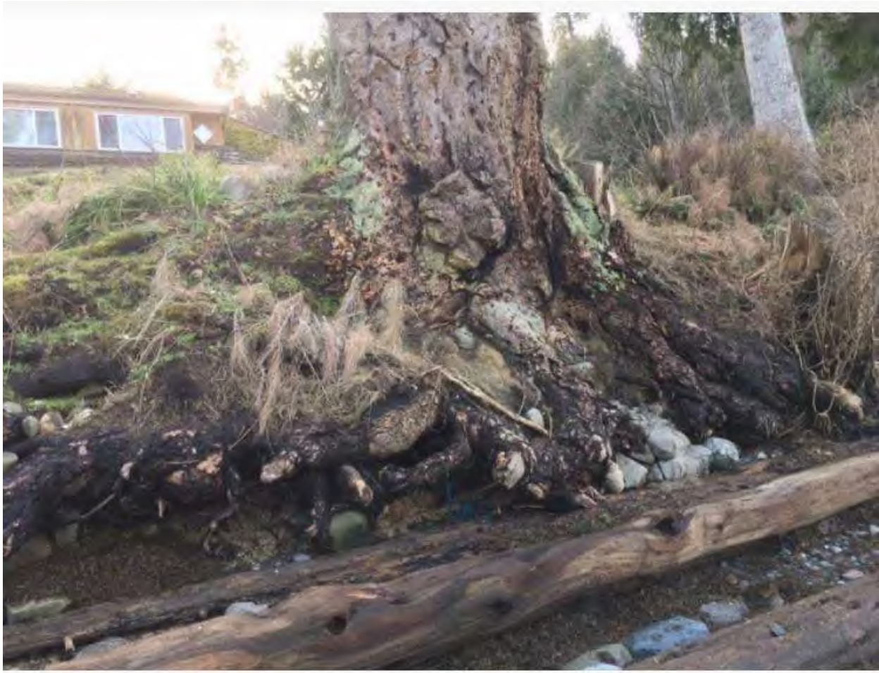
Fig. 4: Exposed roots of D. Fir @ subject property, prior to breakwater installation
