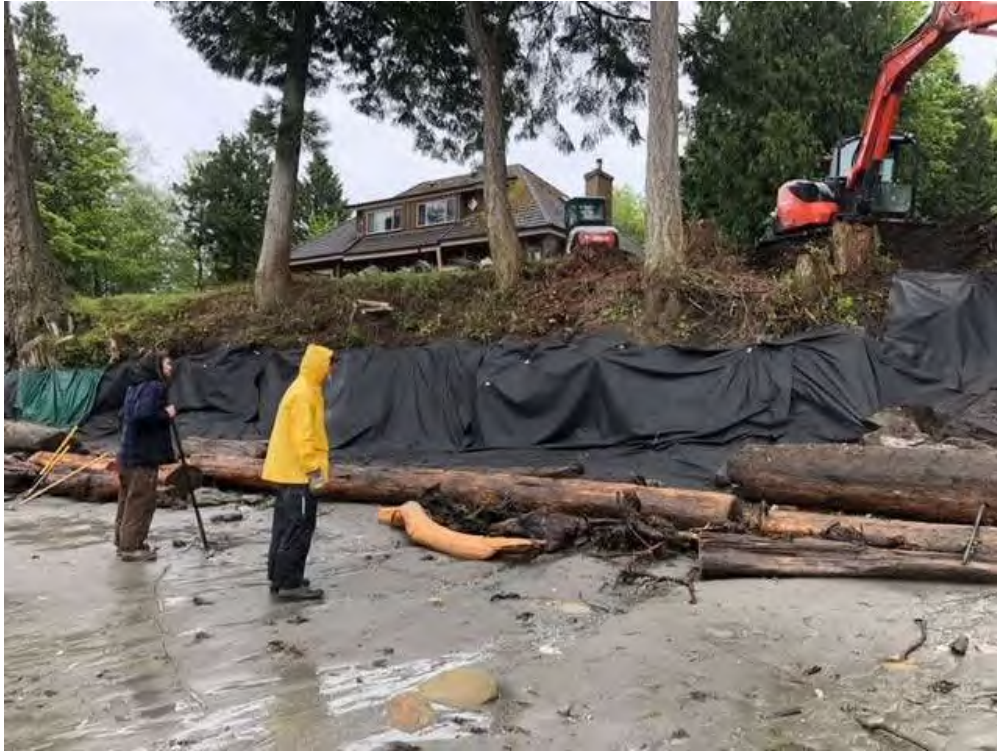
Figure 3.1 Revetment Installation on Steep Eroded Bank
