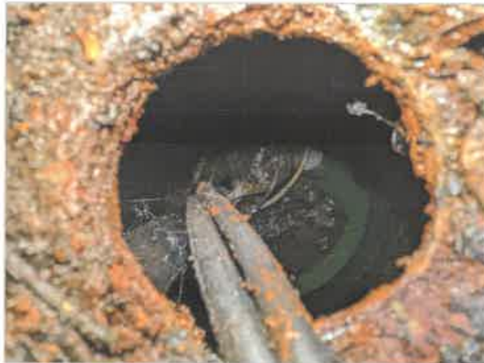
Picture 4: Camera view inside lift station
