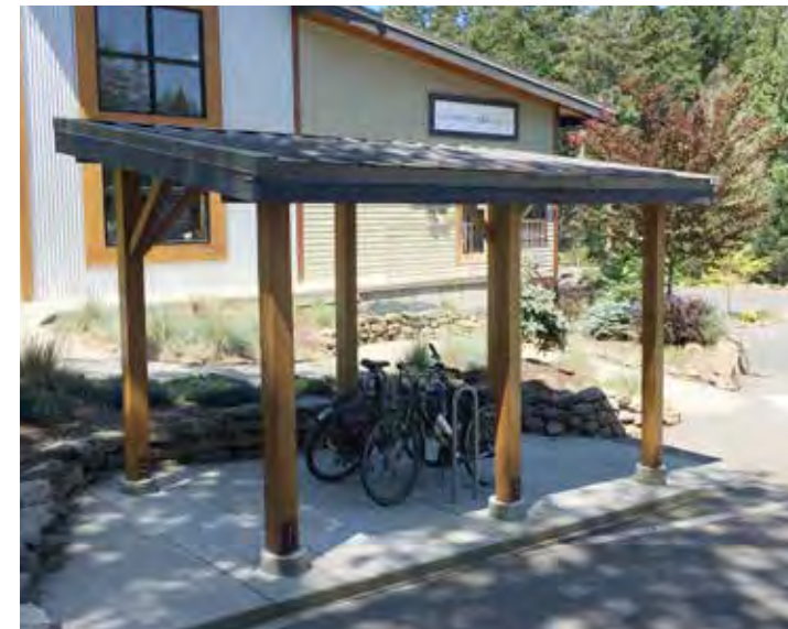
Figure 23: Install a covered bike stand at the terminal given the high numbers of cycle commuters using the terminal
