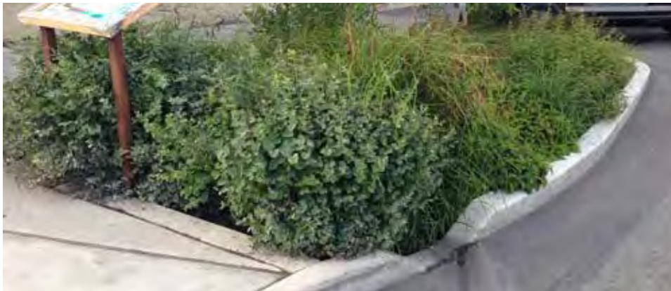
Figure 24: Implement sustainable storm water bioswales/rainwater gardens to deal with storm water run-off where possible
