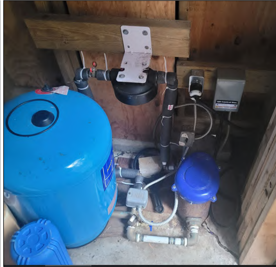
Photograph B1 (LEFT): Looking north towards the pumphouse on Lot A. Photograph B2 (RIGHT): Looking down and inside the pumphouse on Lot A at WTN 26181. The pressure tank, in-line filter and wellhead are shown.
