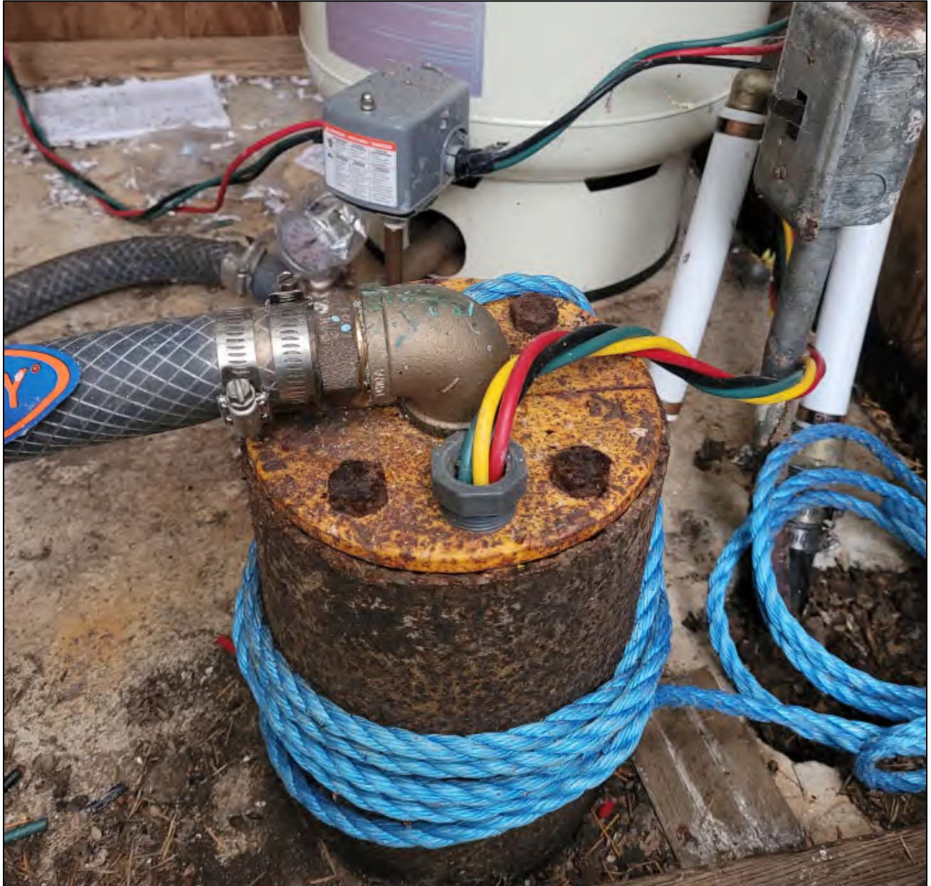
Photograph B5: Close up of the WTN 26180 wellhead. The wellhead cap could not be lifted without removing the pump, which would require assistance from a pump installer.
