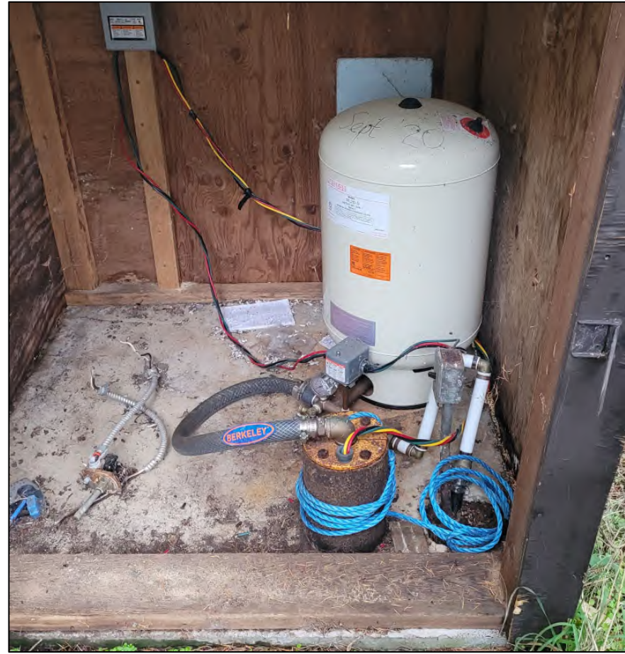
Photograph B3 (LEFT): Looking north towards the pumphouse on Lot B. Photograph B4 (RIGHT): Looking down and inside the pumphouse on Lot B at WTN 26180. The pressure tank and wellhead are shown
