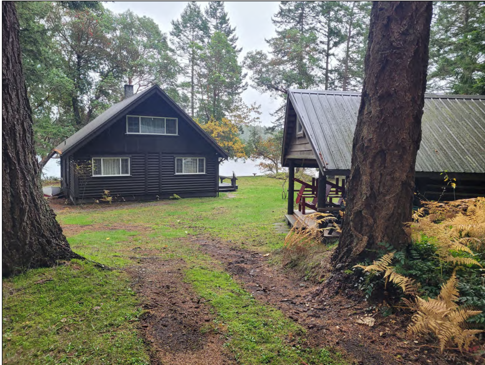
Photograph B6: Looking east at Lot A cabin and the coastline. Topography is sloping from west to east towards the ocean.
