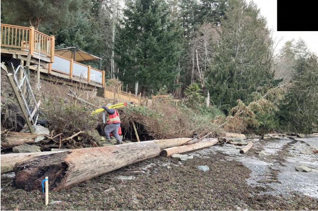
2.) Looking west from NE corner at eroding bank
