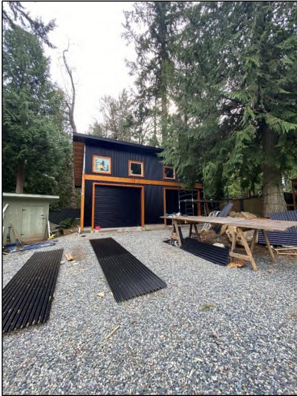
BUILDING LOCATION – LOOKING SOUTH
