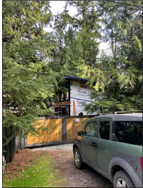
BUILDING LOCATION – LOOKING SOUTH-EAST FROM CANSO RD.
