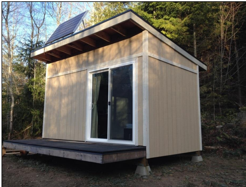
Picture 3: Newly constructed meditation hut on Lot A
