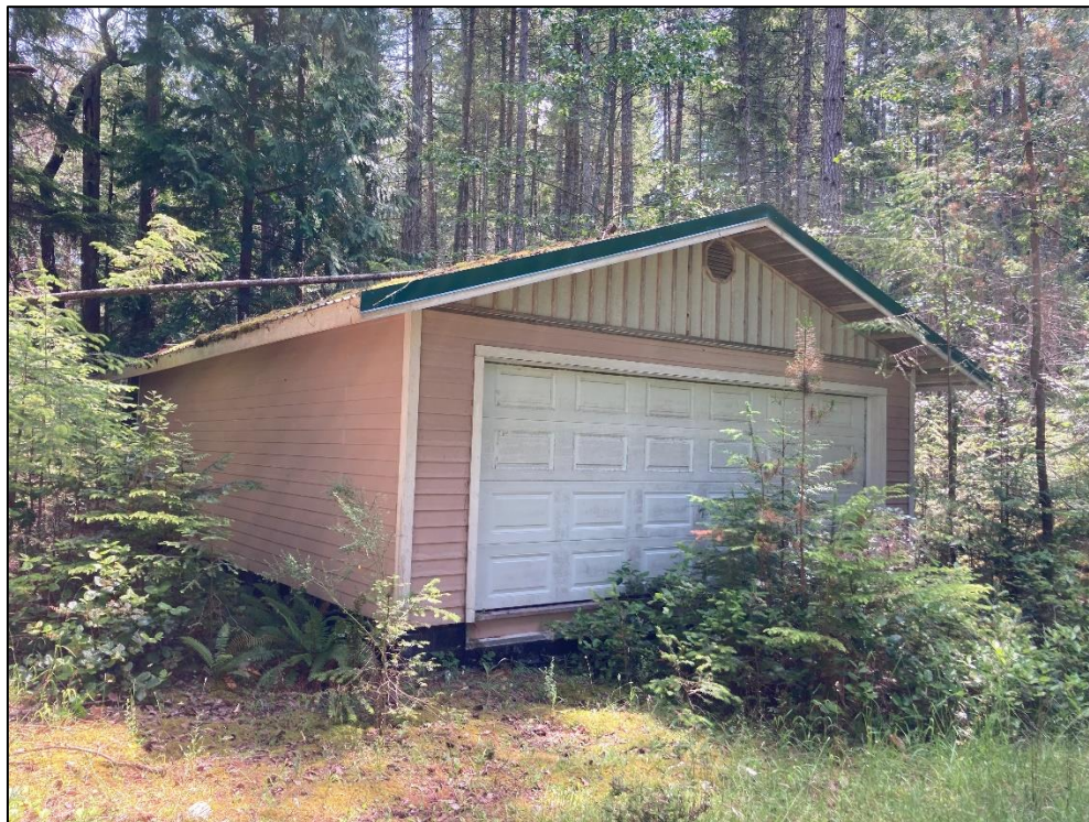
BUILDING (WITH NO POWER OR WATER)
