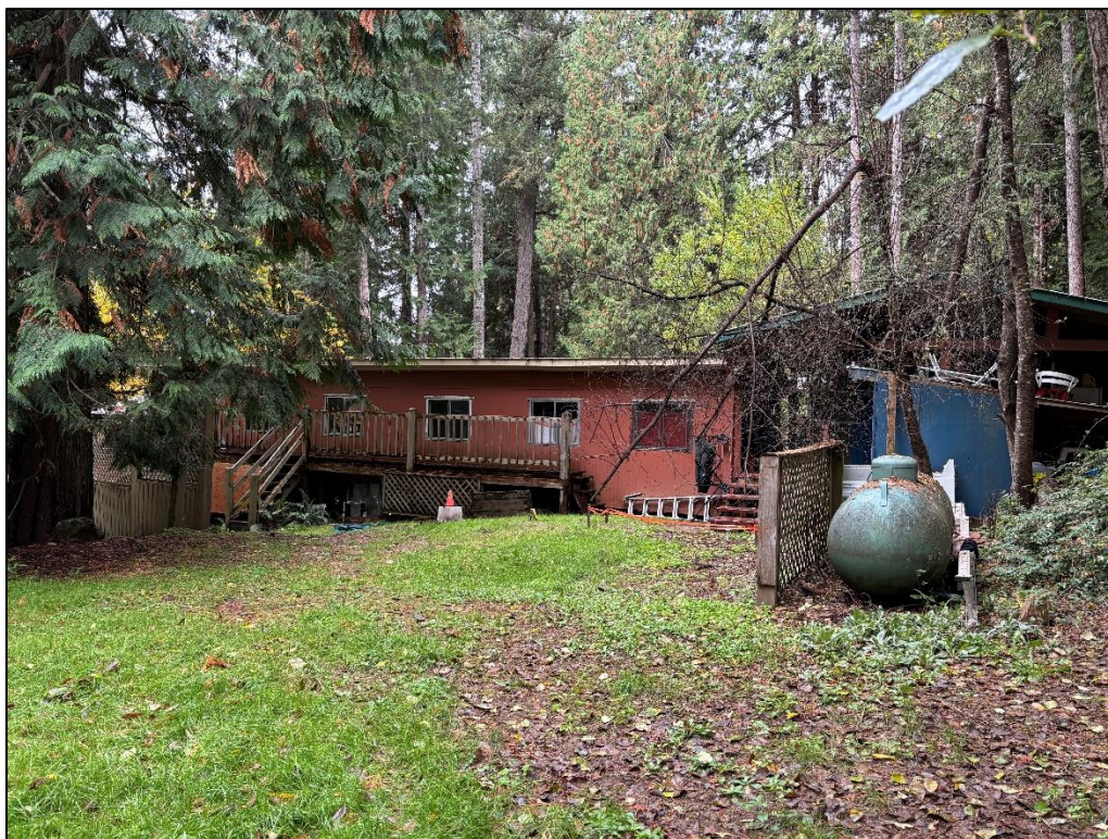
LOOKING WEST TOWARDS EXISTING BUILDING
