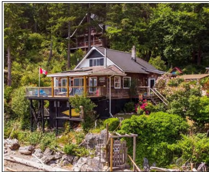
Figure 1 - View from foreshore, secondary dwelling background
