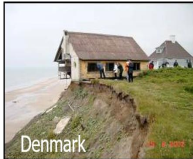
Poor Site Planning
