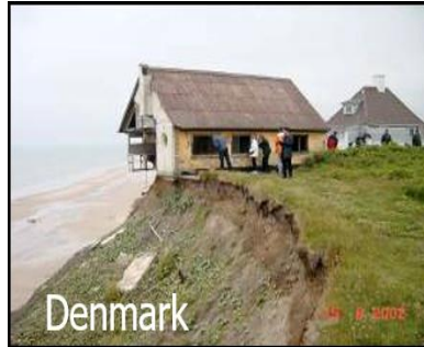
Poor Site Planning
