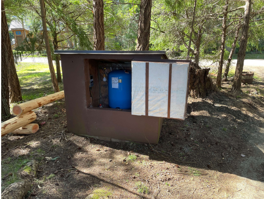
Photo. 5 Well house on the Property.
