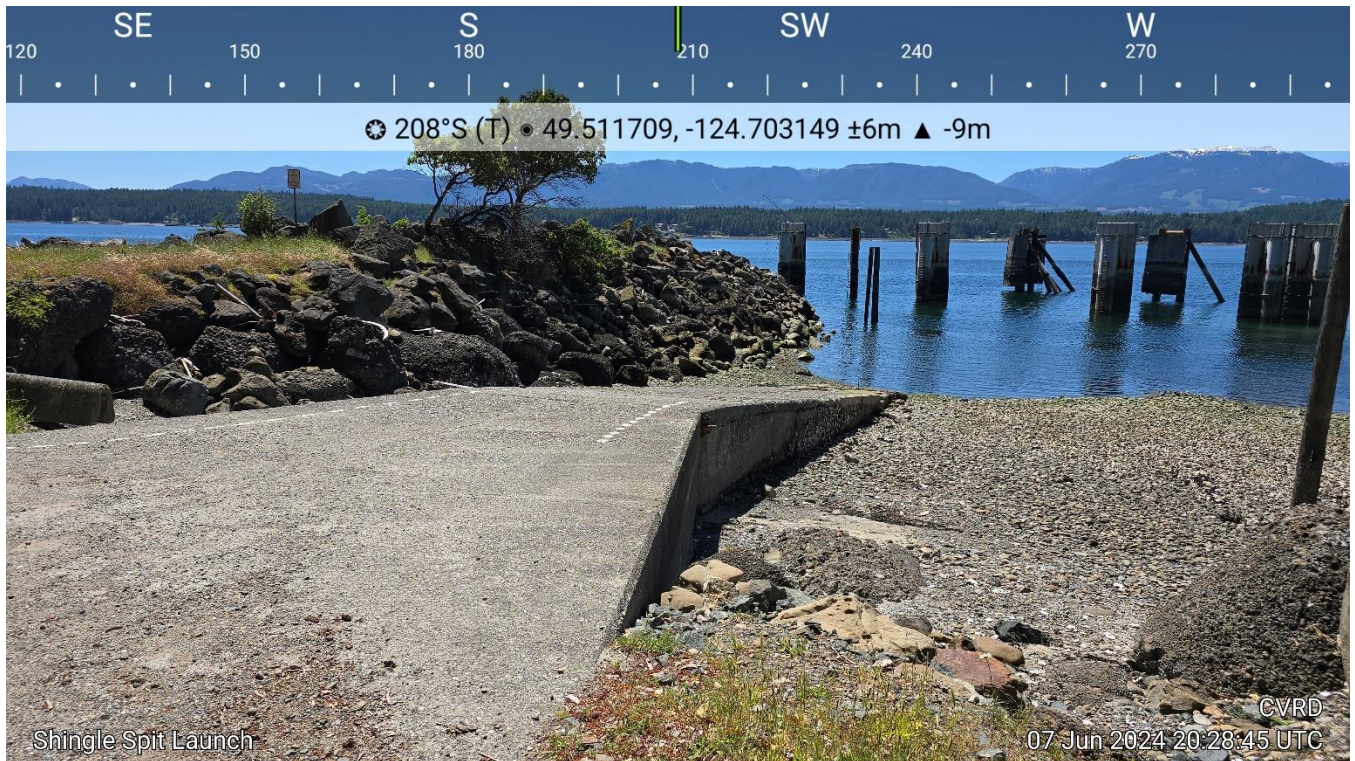
Photo 5. Showing position of the launch in relation to the breakwater and BC Ferry Dock (background, at right).
