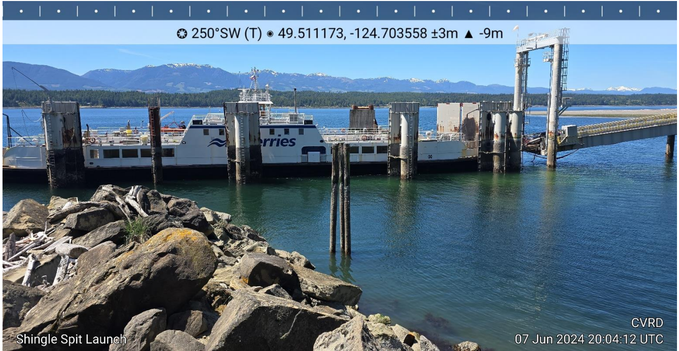
Photo 7. Showing the BC Ferry at dock directly in front of where the new launch is going to be placed, as viewed from the breakwater (foreground, at left).
