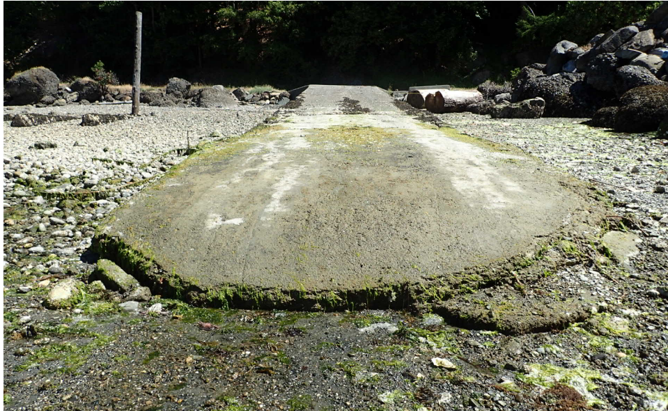
Figure 12 – View of Bottom End
