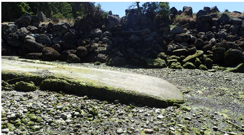
Figure 13 – View of Bottom End Right Side and Water Flow
