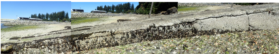
Figure 9 – South Side of Ramp
