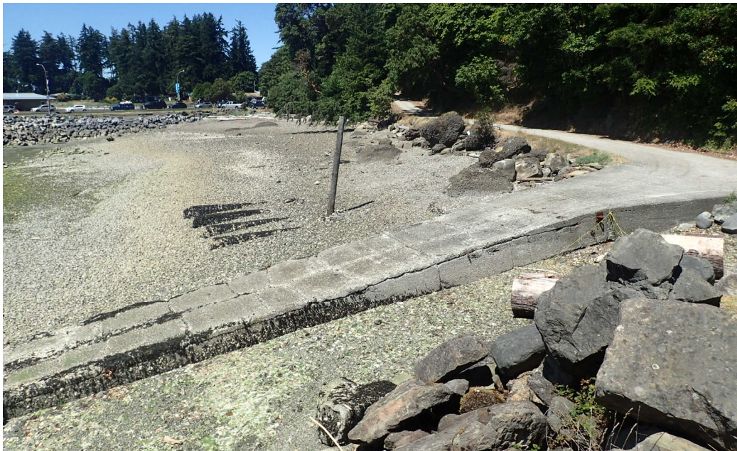
Figure 1 – View of Ramp Towards Ferry
