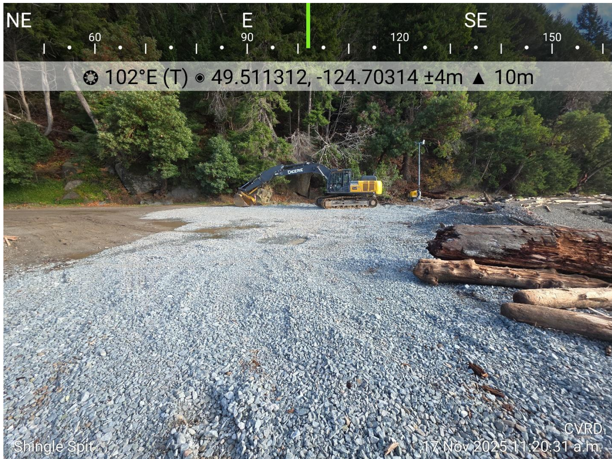
Photo 1. Blast rock has been spread across the landing area just south of the boat launch, The material appears clean and likely inhibits erosion and sediment generation. The Deere 300 excavator in the background is not associated with this project. Ownership of the light plant is not known.
