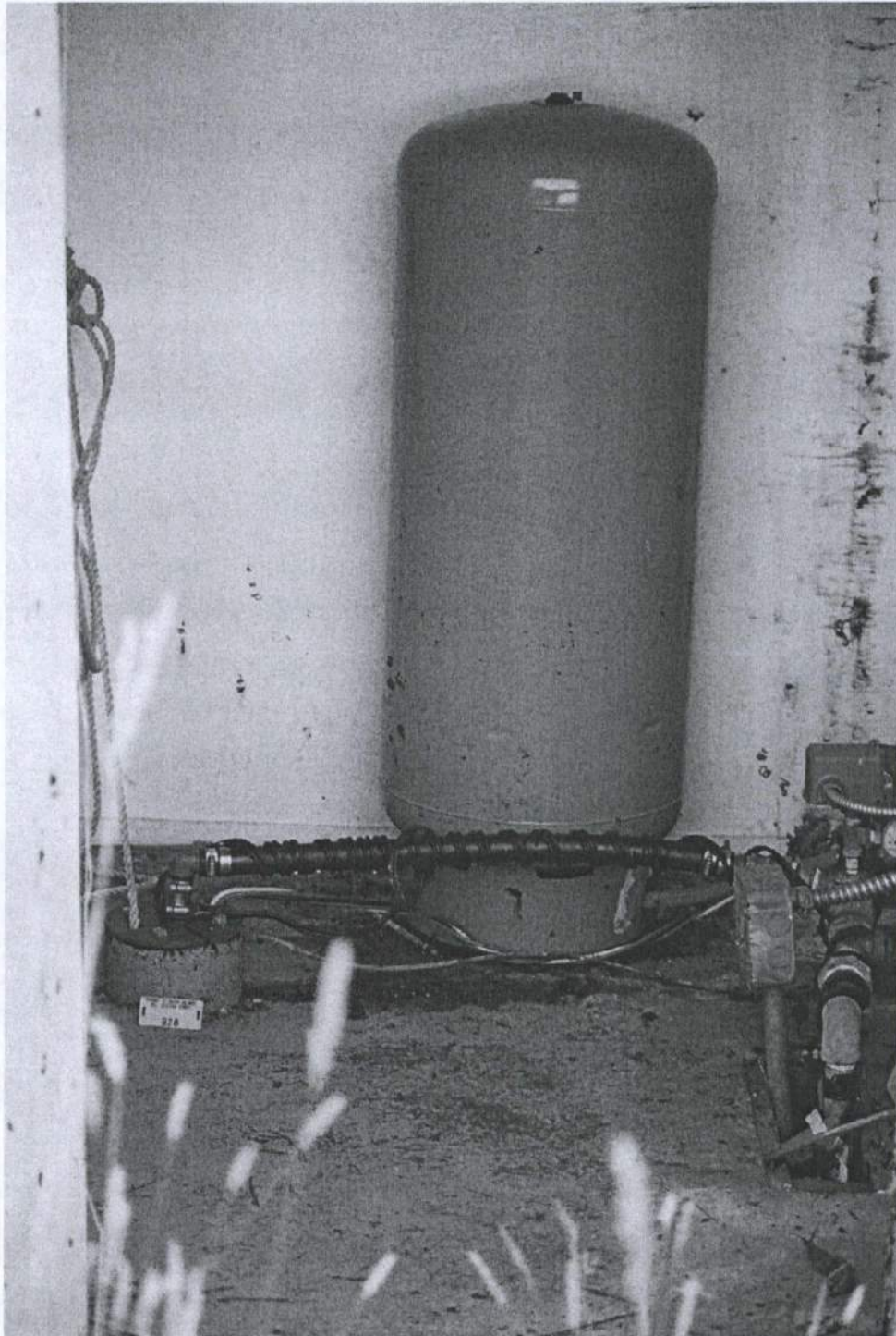
Photo 3: Well and pumphouse interior.
