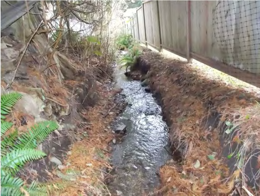
Looking downstream at the channel morphology of the East Fork of the drainage. Note the straight channel and excavated sidewalls, which are typical of ditches.
