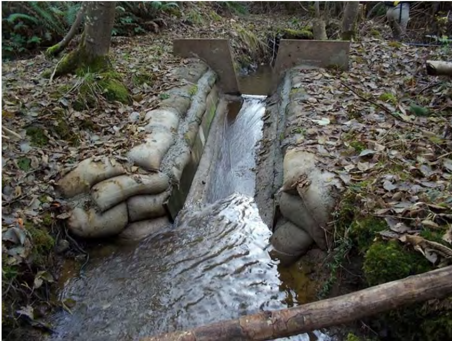
Looking south at a dam system that was likely installed for the purpose of retaining water in particular areas of the stream to provide a water source for residential use.
