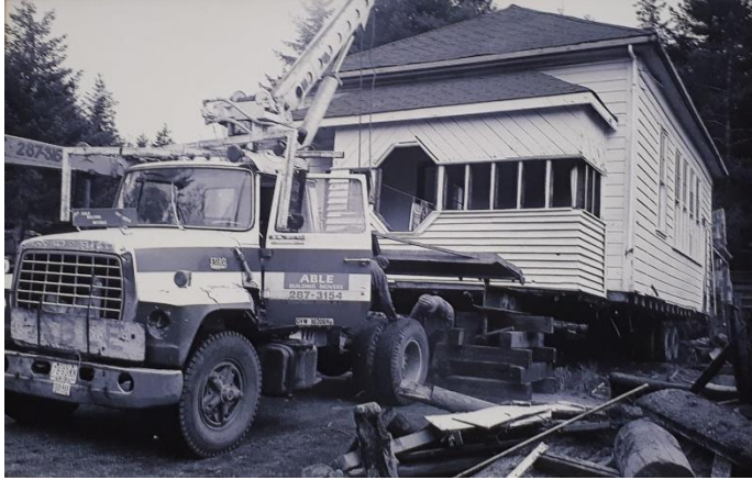
Figure 5. Relocating the Old Schoolhouse with truck, 1984. The 1972 modifications (front entry and windows) are clearly visible. Hornby Island Archives/New Horizons Collection.
