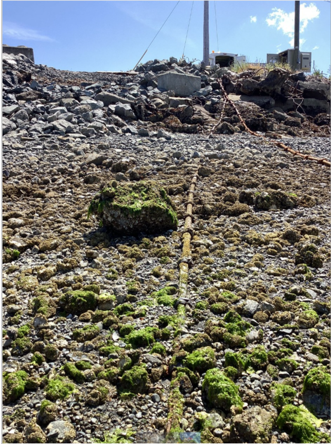
Connected Coast installation adjacent to the Barge ramp at Nanoose Bay which is adjacent to a concrete boat ramp and rock wave barrier
