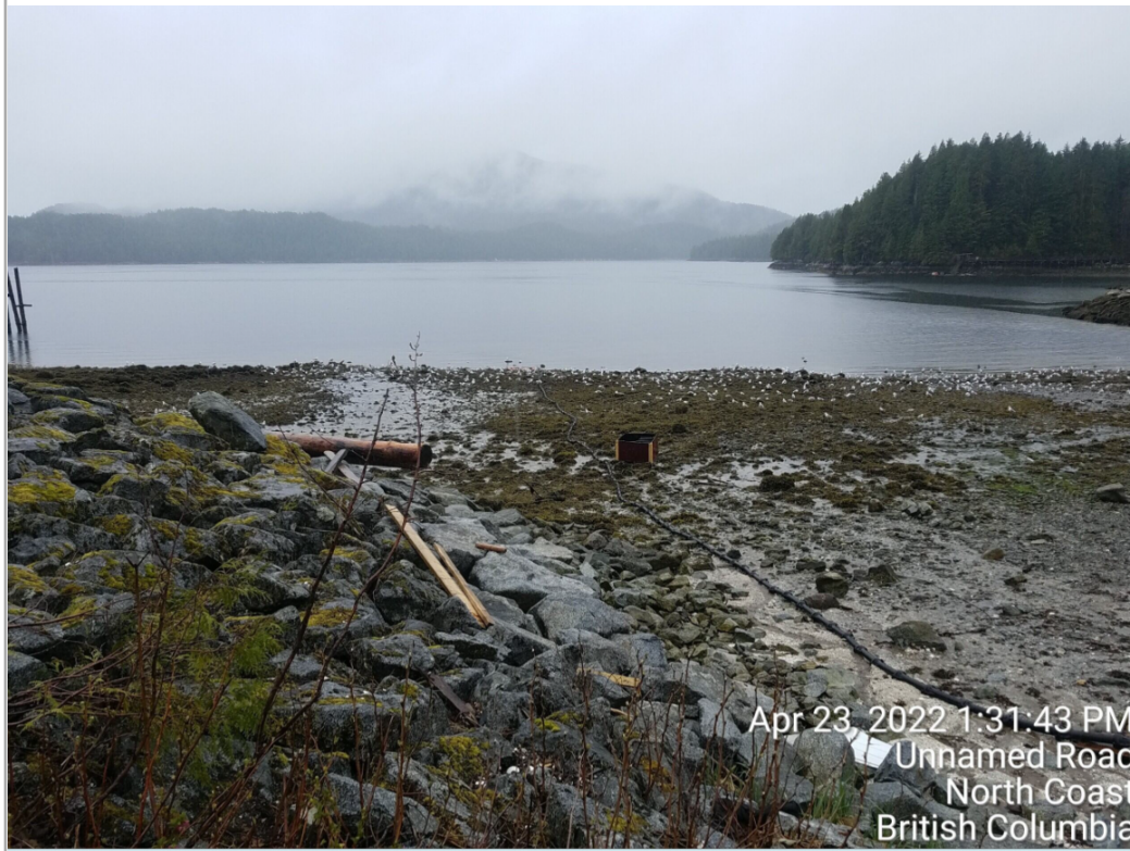
Connected Coast Installation adjacent to the Hartley Bay Barge loading area
