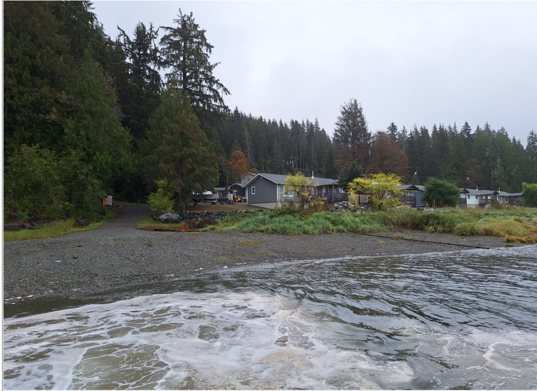
Connected Coast Installation at Uchucklesah t adjacent to the community's boat launch, this community is exclusively boat access.
