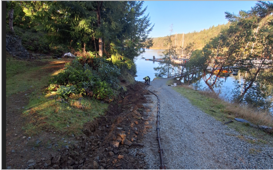
Split pipe construction at Musgrave Landing Boat Ramp
