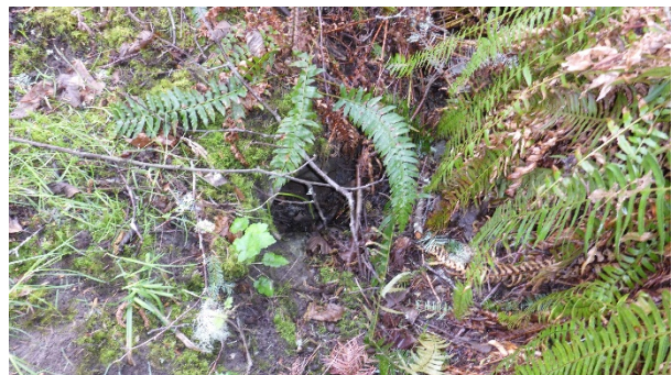
Photo 18. Inlet to West culvert.
