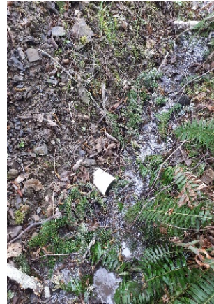
Photo 14. Upstream end of North culvert and surrounding habitat.
