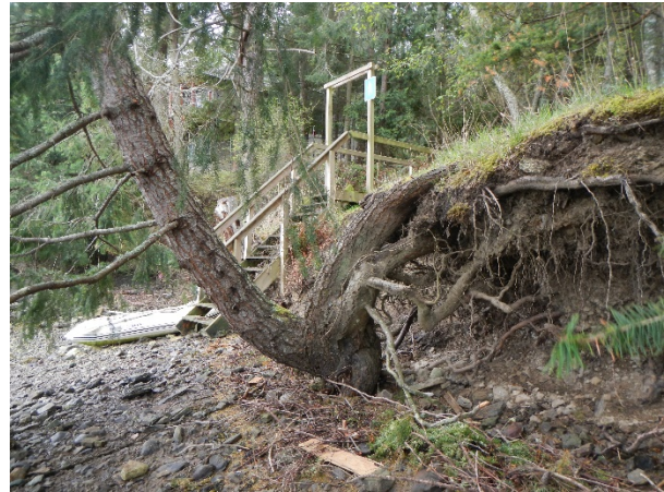
Photo 2. View east from head of transect, showing overhanging Douglas fir eroded roots and current staircase for shore access from Anson Road.
