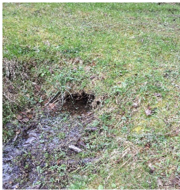
Photo 15. Outlet of East culvert.
