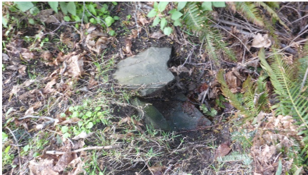
Photo 21. Concrete culvert at top-of-bank that runs under Horton Bay Road.
