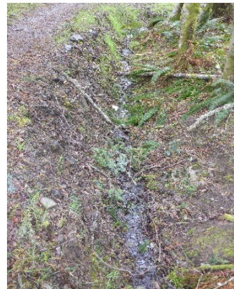
Photo 10. Ditch running along dirt driveway, leading to Northwest culvert.
