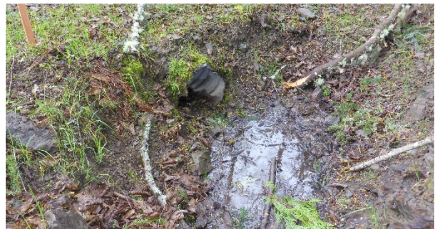
Photo 12. Entrance to Northwest culvert.
