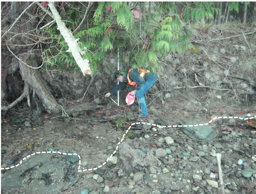
Figure 6. A photo of the cliff base near the 35-m mark. The dotted line indicates the approximate seaward limit of the stiff clay outcrop that occurs near the “nose” of the Anson Rd right-of-way.
