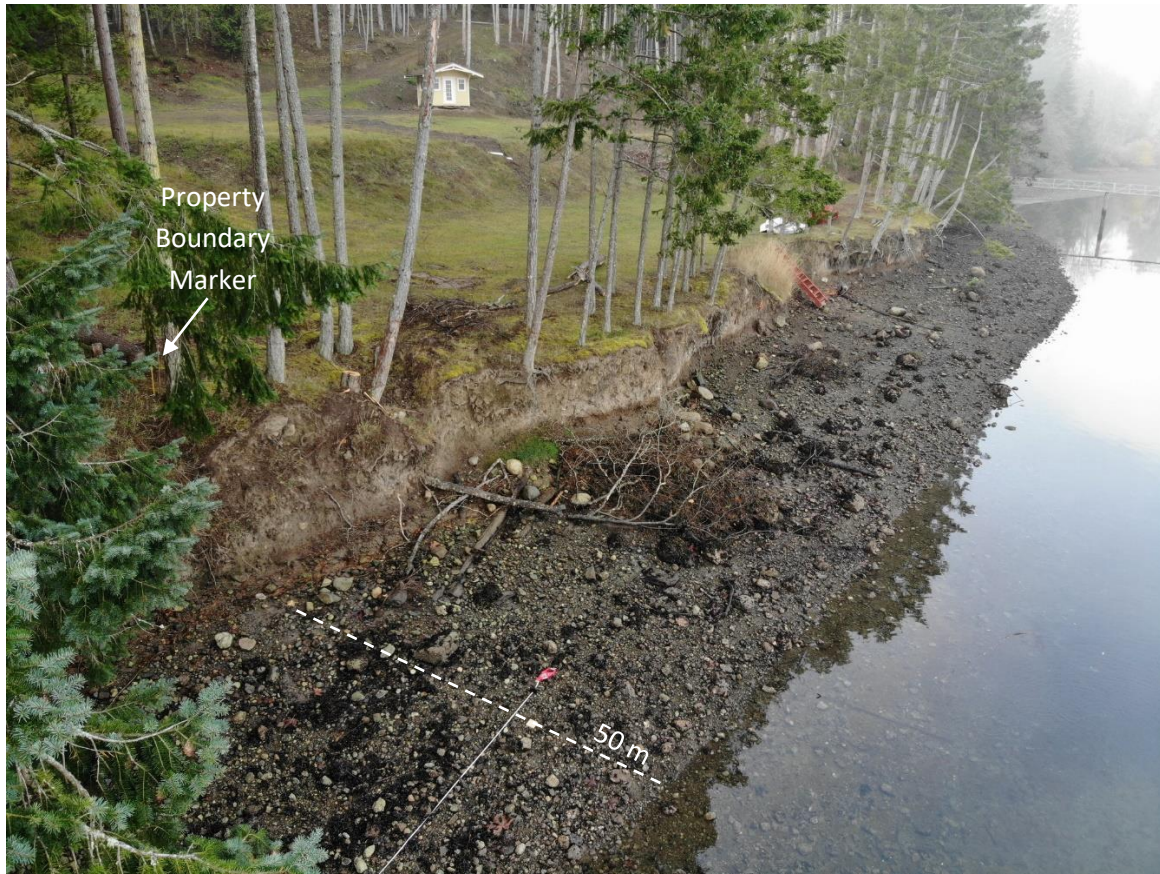
Figure A-6. Drone photo of Section 50-m looking west.
