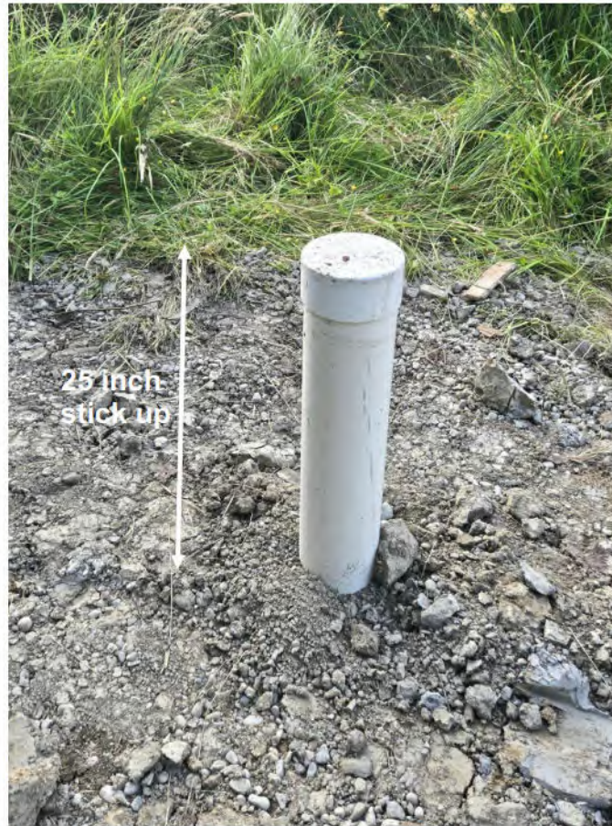
Photo 9. Completed 6 inch diameter monitoring well, June 30, 2025.
