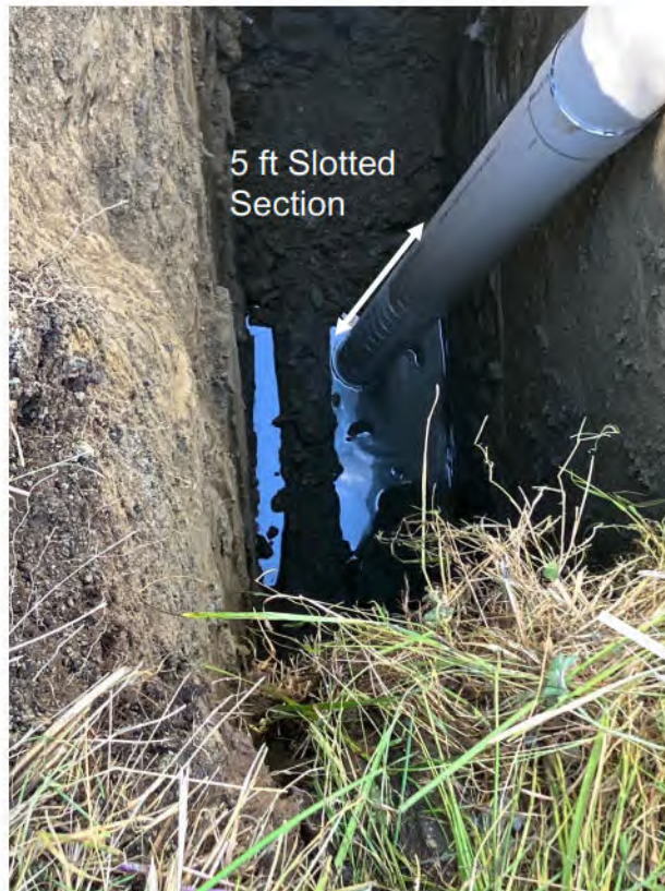
Photo 5. Monitor well casing set in excavation. Note water in bottom of excavation, June 30, 2025.
