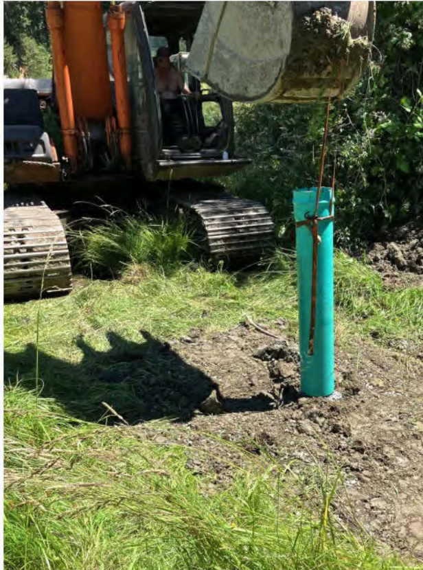
Photo 8. Pulling out 8 inch temporary surface casing, June 30, 2025.
