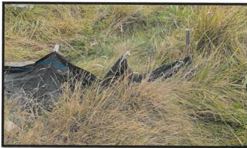
Photo 10: Silt fencing down gradient from operations area, required maintenance prior to rainy season.
