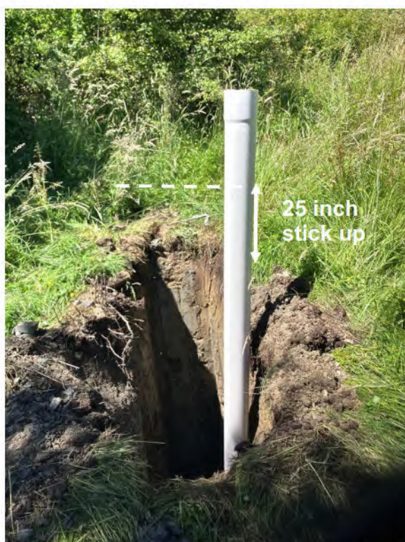
Photo 4. 6 inch diameter PVC well casing set in excavation to depth of 15 feet (4.6 m), June 30, 2025. Casing was subsequently cut to provide a 25 inch (63.5 cm) stick up above ground level.
