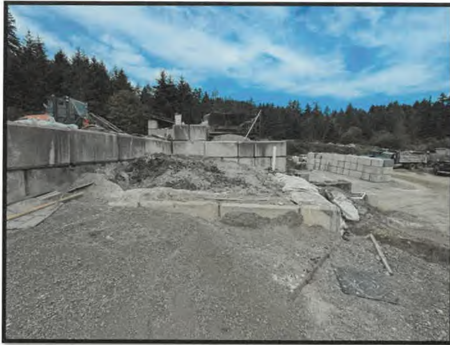
Photo 5: Solids storage area
