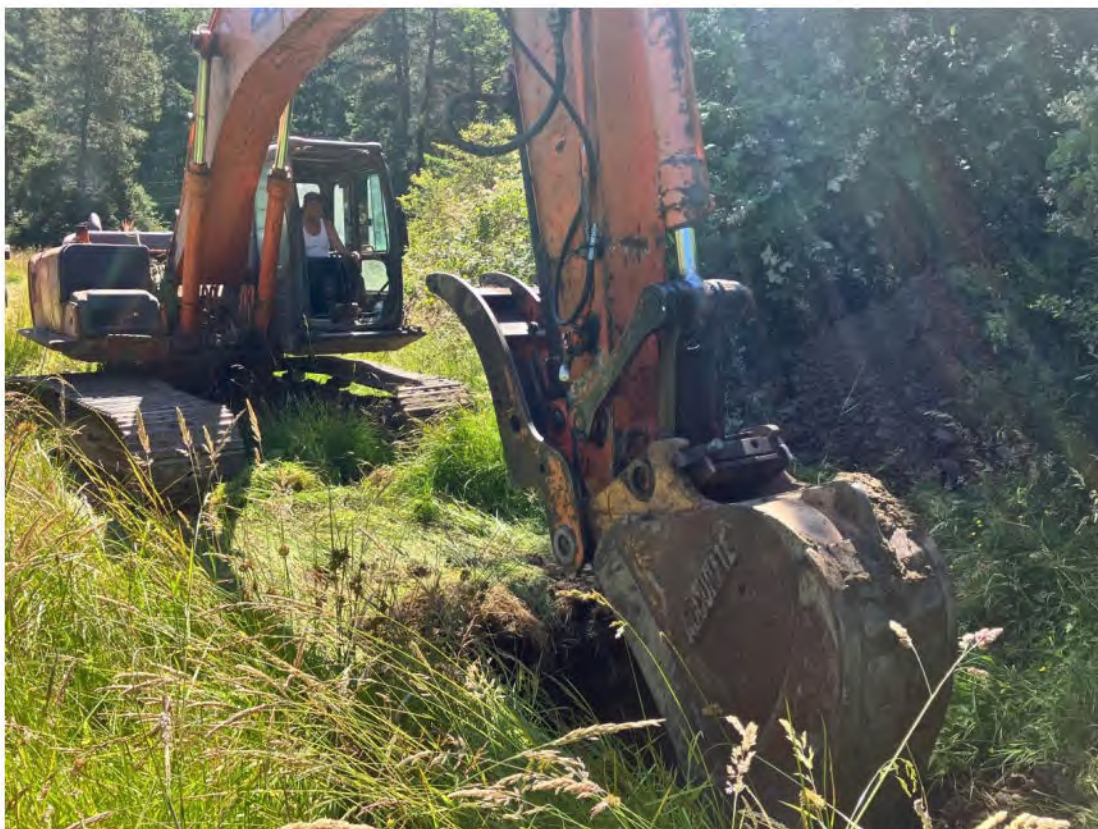
Photo 1. Excavator employed to install monitor well, June 30, 2025.
