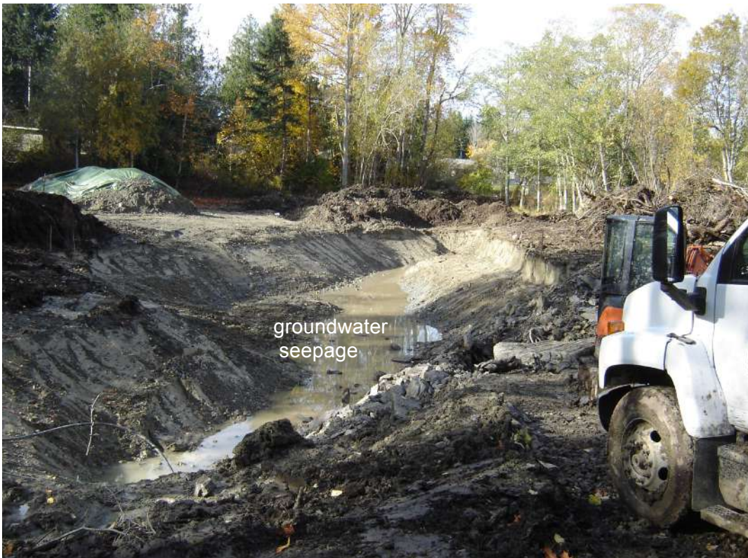
Photo 2. Excavated pond looking westerly, late summer 2008. Note groundwater seepage into pond.
