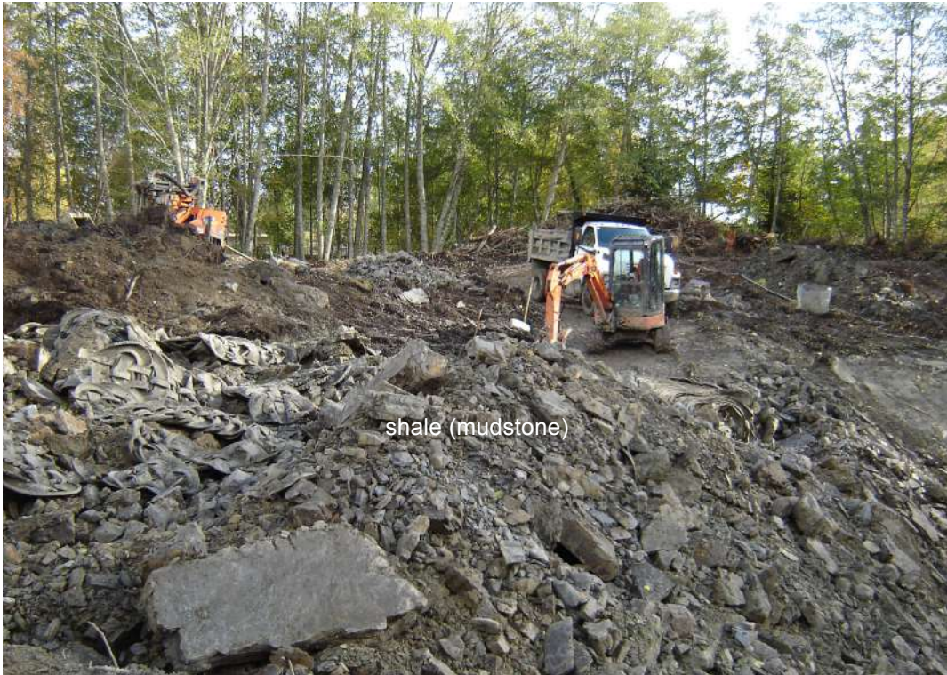
Photo 1. Shale (mudstone) bedrock, blasted and excavated late summer 2008, photograph looking northeasterly.
