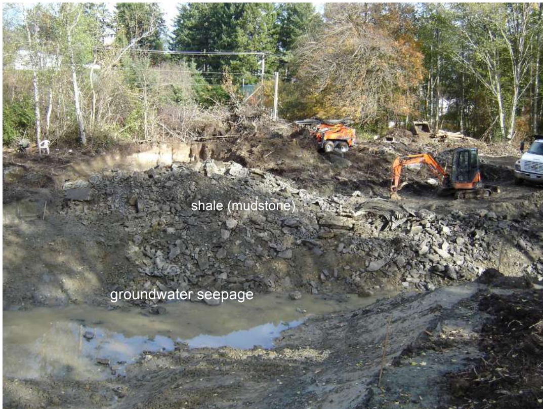
Photo 4. Shale (mudstone) bedrock exposed in excavation, late summer 2008. Photograph looking northeasterly.
