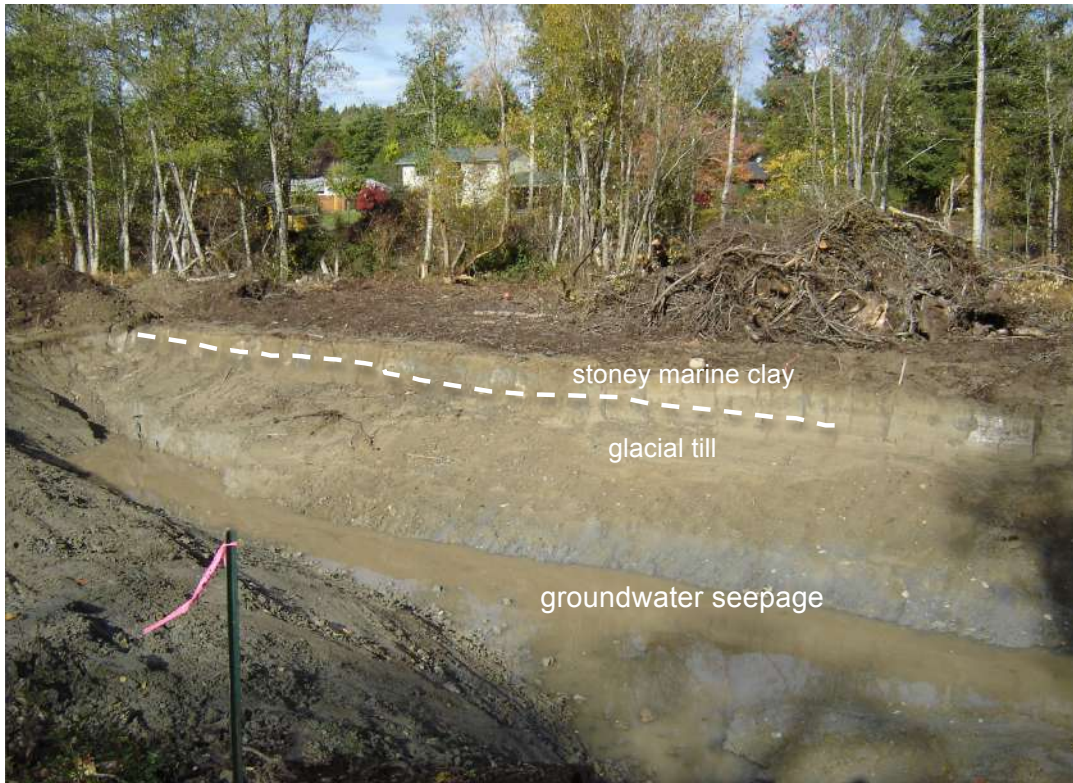
Photo 3. Excavated pond looking northerly showing exposed stoney marine clay overlying glacial till, late summer 2008.
