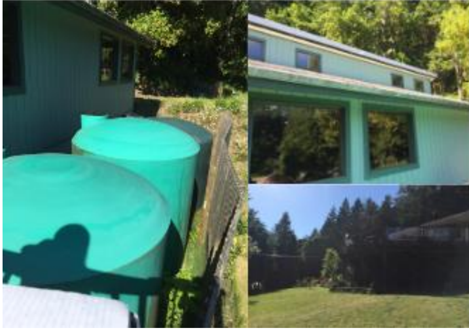
Figure D5. Case study C2 images taken by Kendra Anderson during site visit May 29, 2017 to gather further details on RWH systems that exist on SSI. Water is collected off the workshop roof and held in three cisterns with a combined volume of 6,600 gallons, used to water the garden area.
