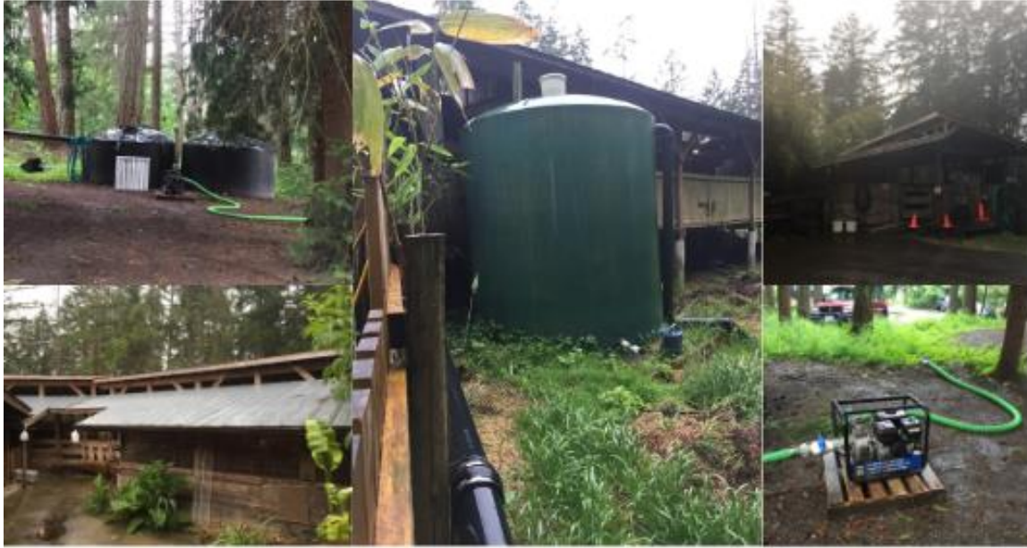
Figure D6. Case study C3 images taken by Kendra Anderson during site visit May 30, 2017 to gather further details on RWH systems that exist on SSI. A 2,100 gallon black cistern is filled from collection off the metal roof and pumped for use in irrigation. The tank was repurposed from previous projects.
