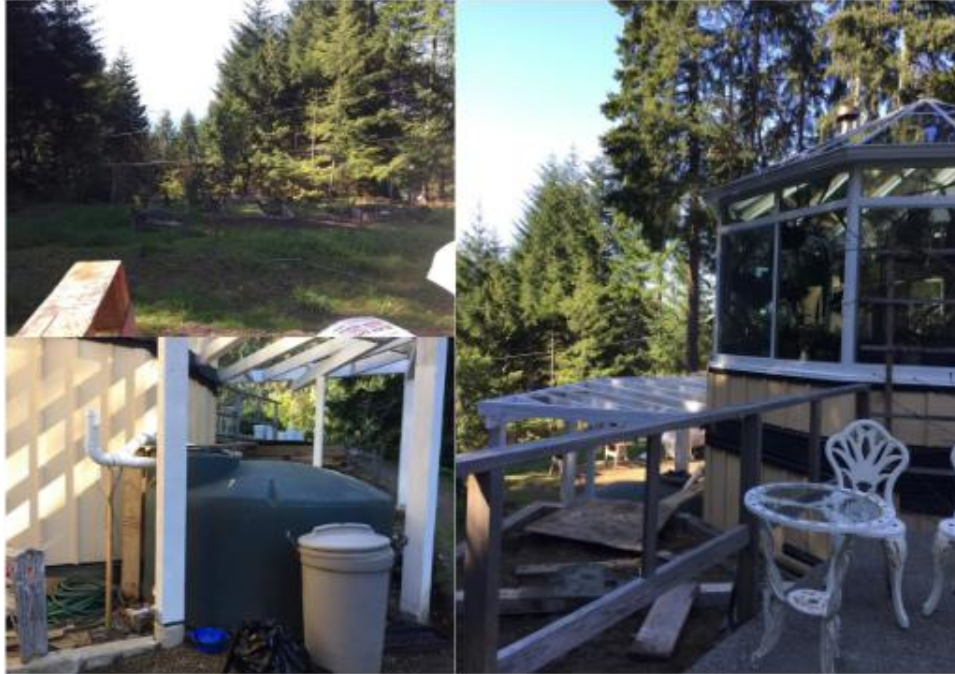
Figure D8. Case study S2 images taken by Kendra Anderson during site visit on April 21, 2017 to gather further details on RWH systems that exist on SSI. Rainwater is collected off the conservatory roof and used on the garden area which is shaded through the afternoon to minimize water use. A 1,100 gallon is used for storage.
